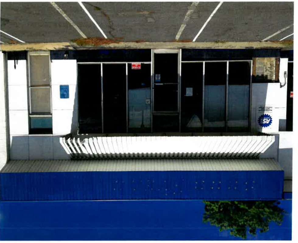
WEST MAIN STREET FACADE
