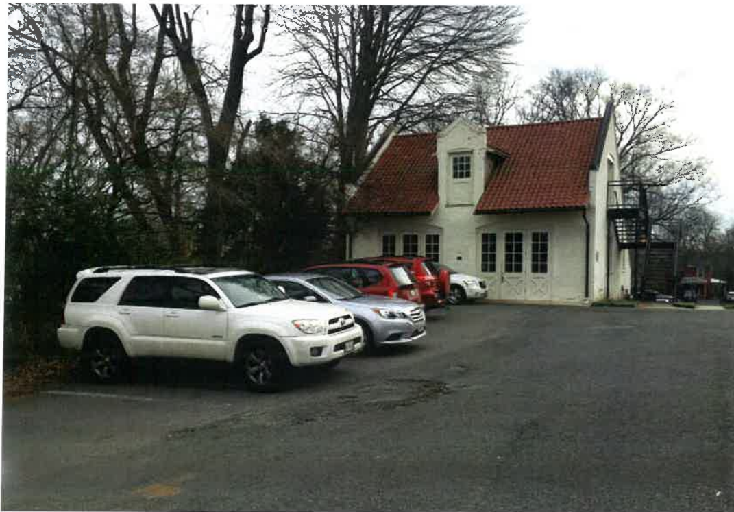
Existing Carriage House
