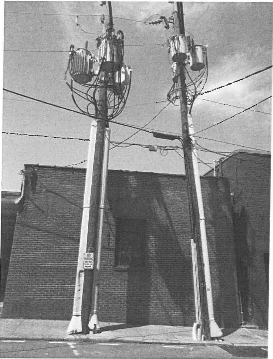
View from 2nd St showing the brick facade, tile coping and painted metal window.
