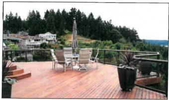
ARS 350 Series Aluminum Railing System With Glass
