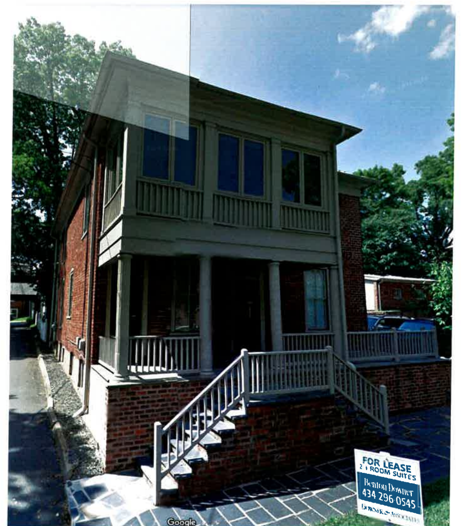
413 7TH ST NE, WEST FACADE
