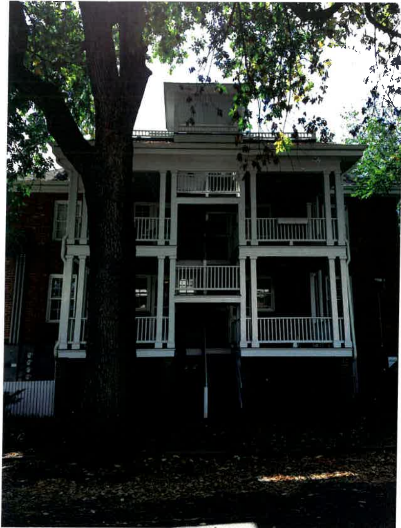
619 EAST HIGH ST, NORTH FACADE
