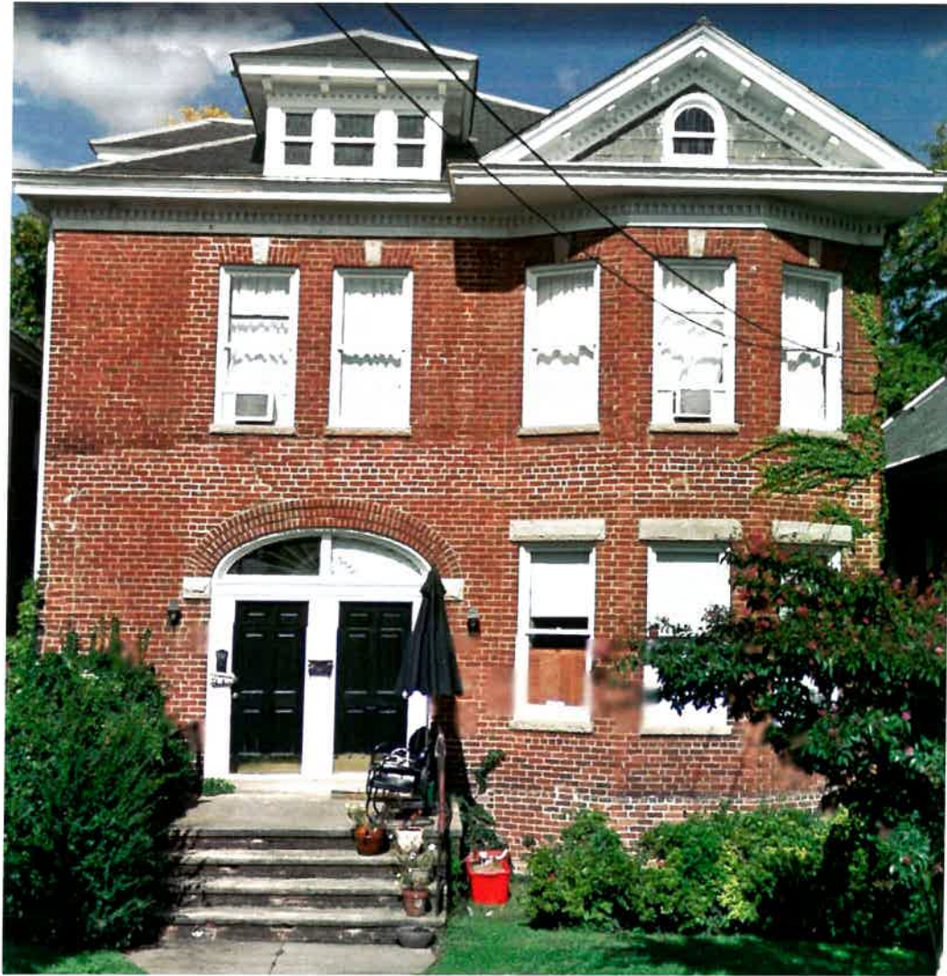
615 E. HIGH ST, SOUTH FACADE
