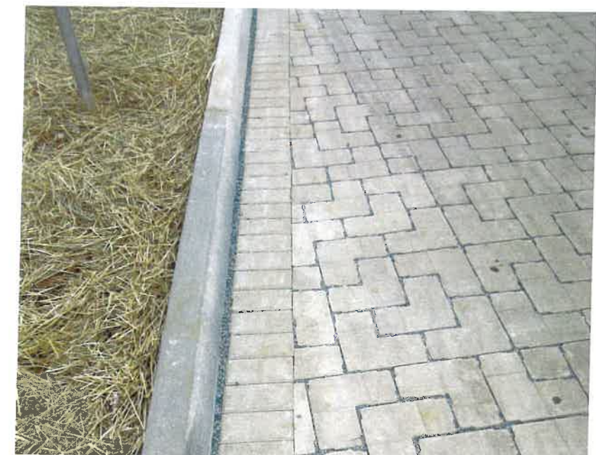
Concrete curb with Eco-Bay James River pavers with edge border pavers. (Note- pavers will be 5x10, not L-shape shown in picture.)
