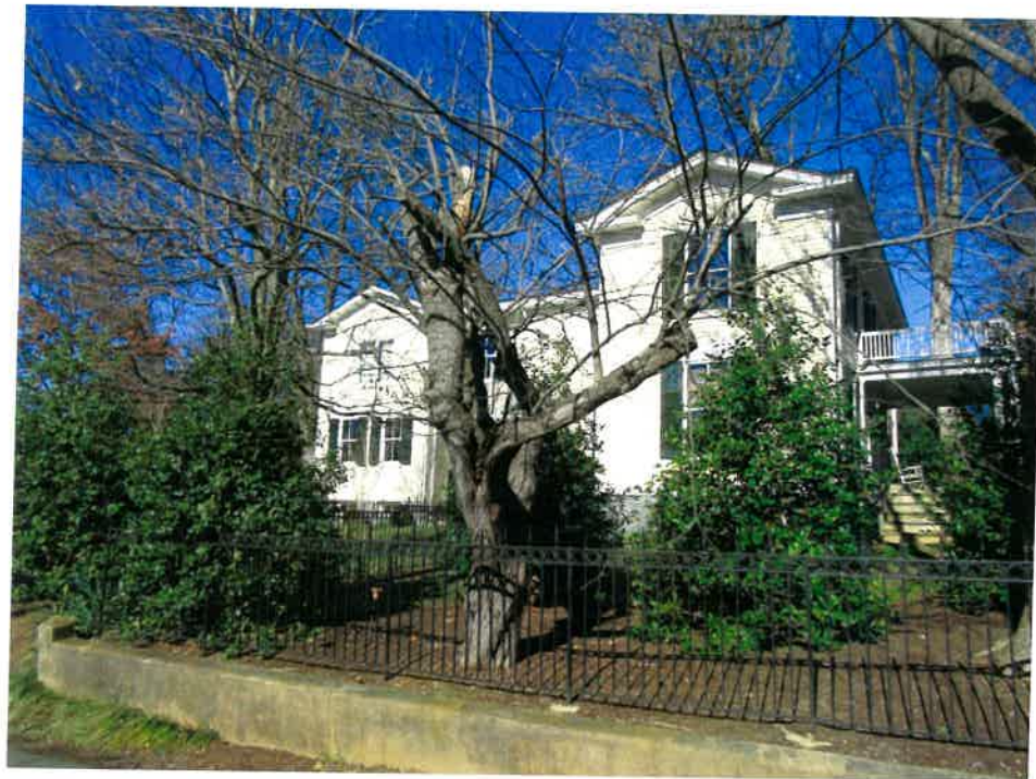
Existing tree to be removed at east entrance
