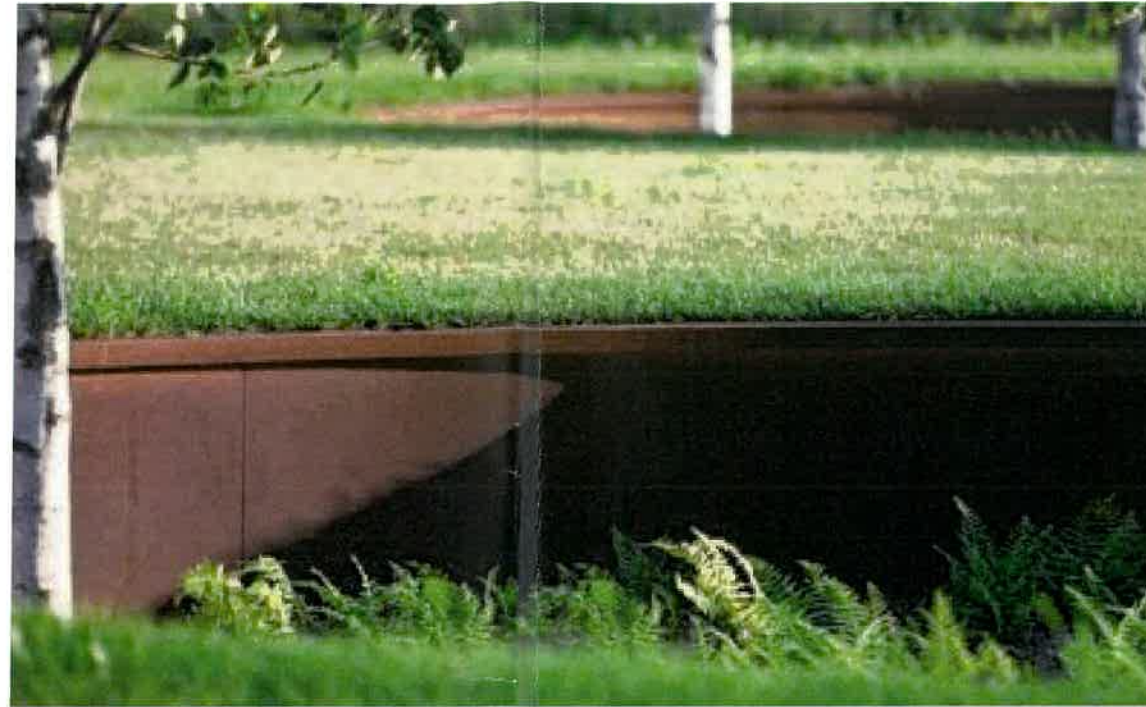
CORTEN STEEL RETAINING WALL
