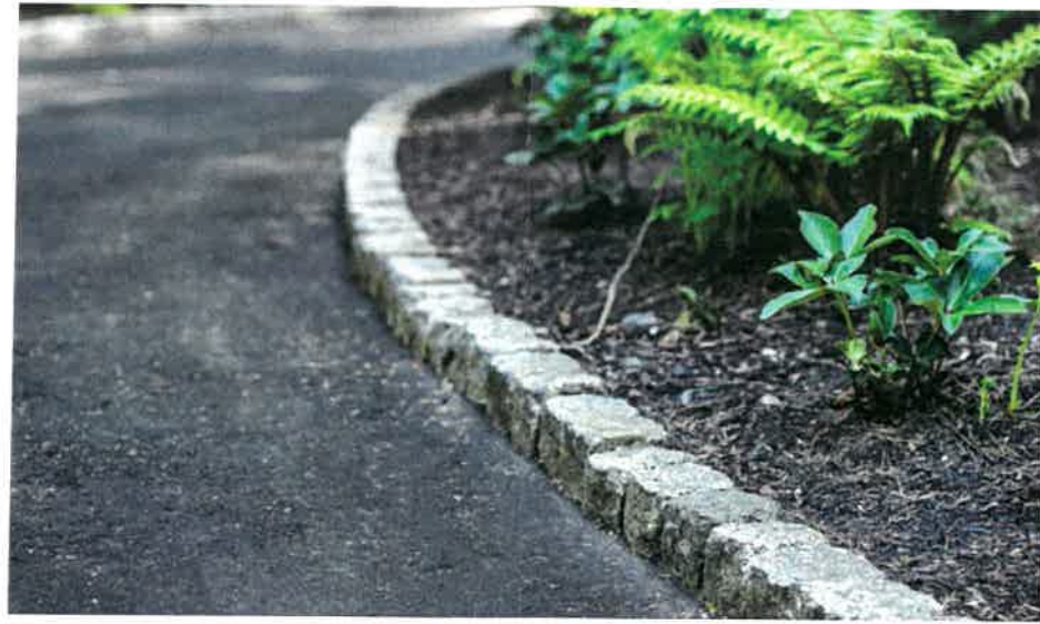
Low Cobble Curb, Asphalt Driveway
