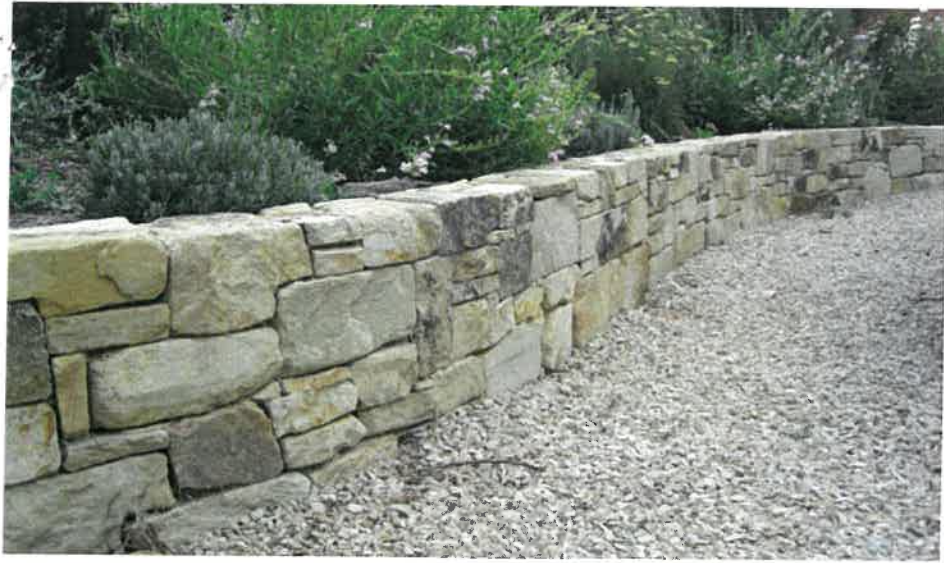
Low Dry-Stacked Stone Wall, Prime & Seal Driveway
