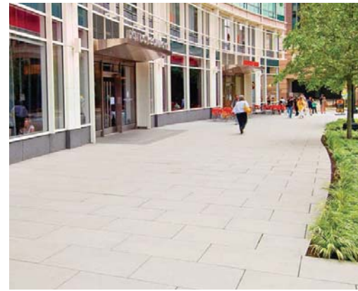
CONCRETE PAVERS - 12"x24"
