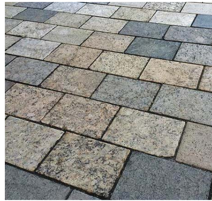
GRANITE PAVERS - 12"x18" WITH THERMAL FINISH
