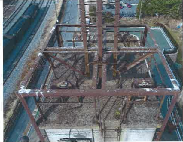
Fig12. Another View of steel on the roof that is being held by rusted chains.
