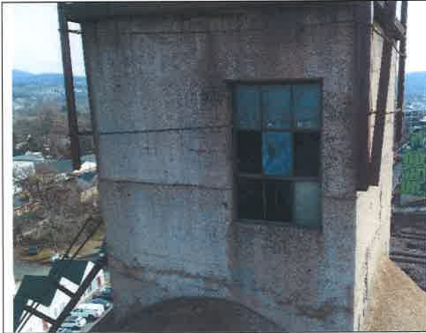
Fig11. View of roof steel that is being held in place by rusted chains.
