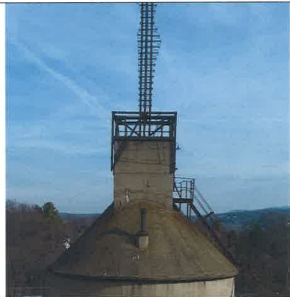
Fig10. SW Roof, vent is to be removed and the hole must be capped. Steel sculpture will be removed.
