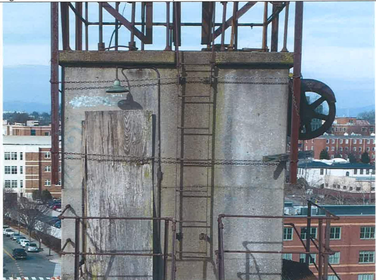
Fig23. View of the top of the tower where the steel is being held on by chains.
