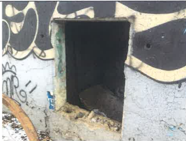
Fig17. View of hole on the wall at the base of the tower. This must be closed off with block and then painted with the rest of the lower portion of the tower.
