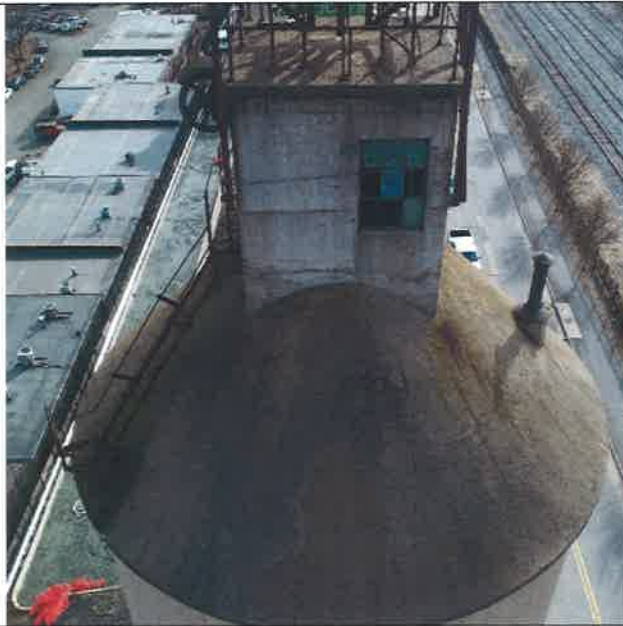
Fig15. Roof on the NW Side of tower. Window is to be replaced. A Charcoal Gray Sealer will be applied to the roof.
