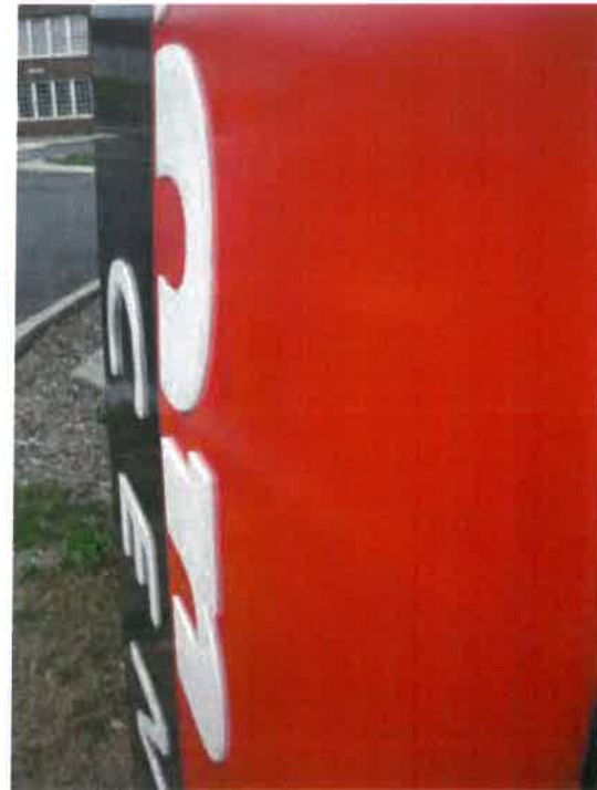
LOCAL EXAMPLE: ALUMINUM CABINET, PUSH THROUGH ACRYLIC CHARACTERS WITH INTERNAL ILLUMINATION. FABRICATED AND INSTALLED BY GROPEN
