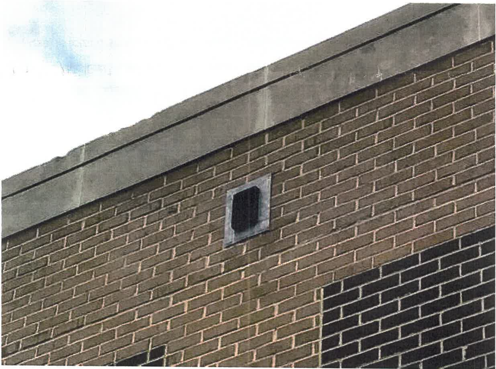
Lewis & Clark existing scupper. New scuppers to be 3" tall by 6" wide, not 8" square as shown above See drawings for detail. New finishes to match existing.
