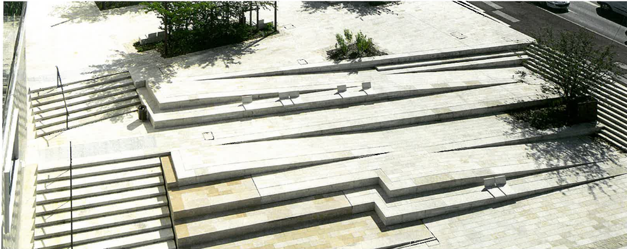
Town Entrance, Ateliers 2/3/4/ · Chatenay Malabry
