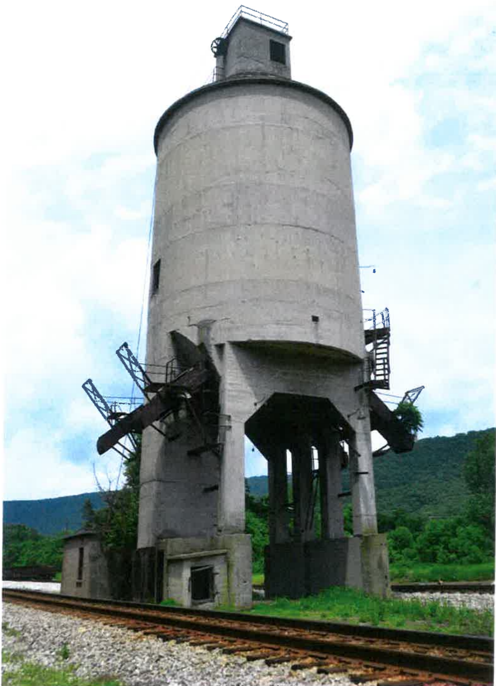
Balcony Falls, VA Coaling Tower with metal components, including coal chutes, still intact.
