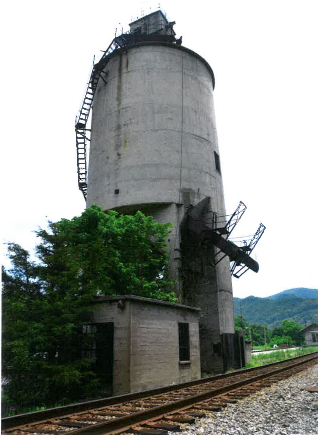
Another view of coaling tower including metal stairs, coal chutes and the structure that housed the engines for operating the coal and sand pulley systems.
