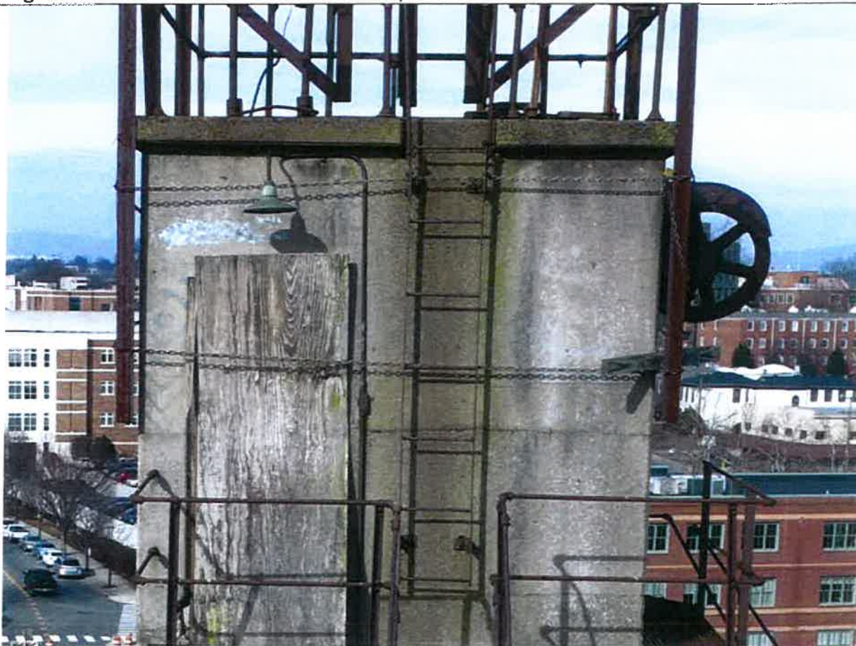
Fig23. View of the top of the tower where the steel sculpture is being held on by chains.
