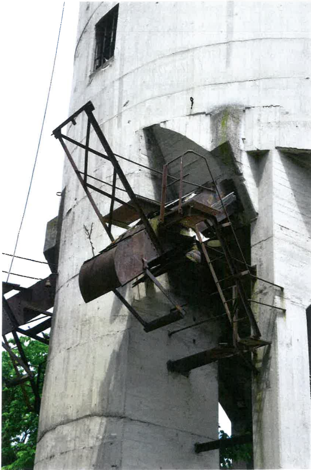
Coal chute apparatus at Balcony Falls. Most metal components were removed from other defunct coal towers and recycled as scrap metal.
