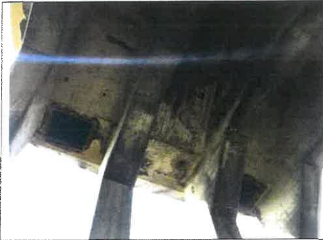
Fig19. View of the holes on the underside of the tower.
