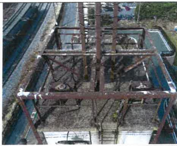
Fig12. Another View of steel on the roof that is being held by rusted chains.
