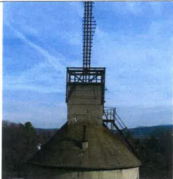
Fig10. SW Roof, smoke jack to be retained. Steel sculpture and stairs will be removed.
