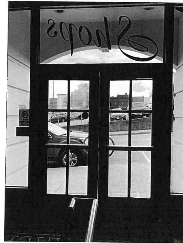
EXISTING WATER STREET ENTRANCE INTERIOR VIEWPOINT
