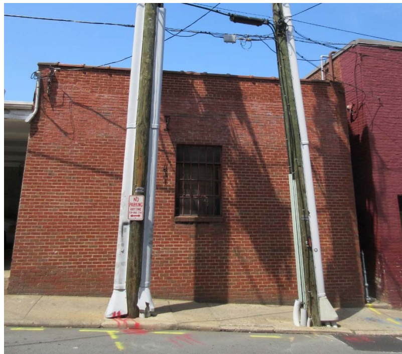
Existing building from Second St
