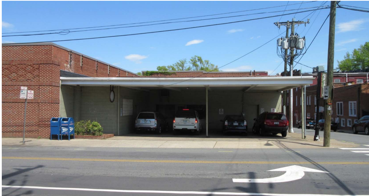
Existing building from Water St
