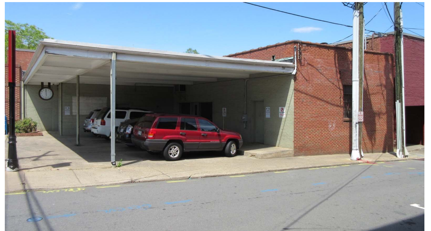
Existing building from Second St
