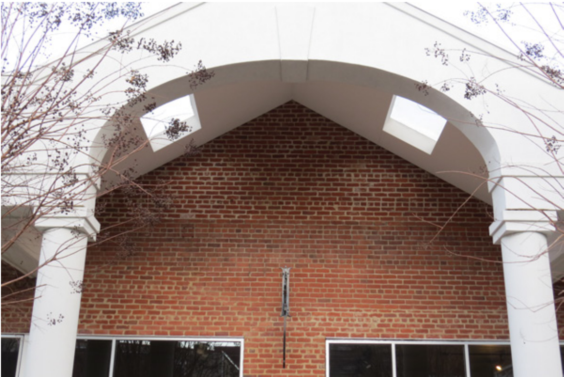
Added brickwork in portico of east façade
