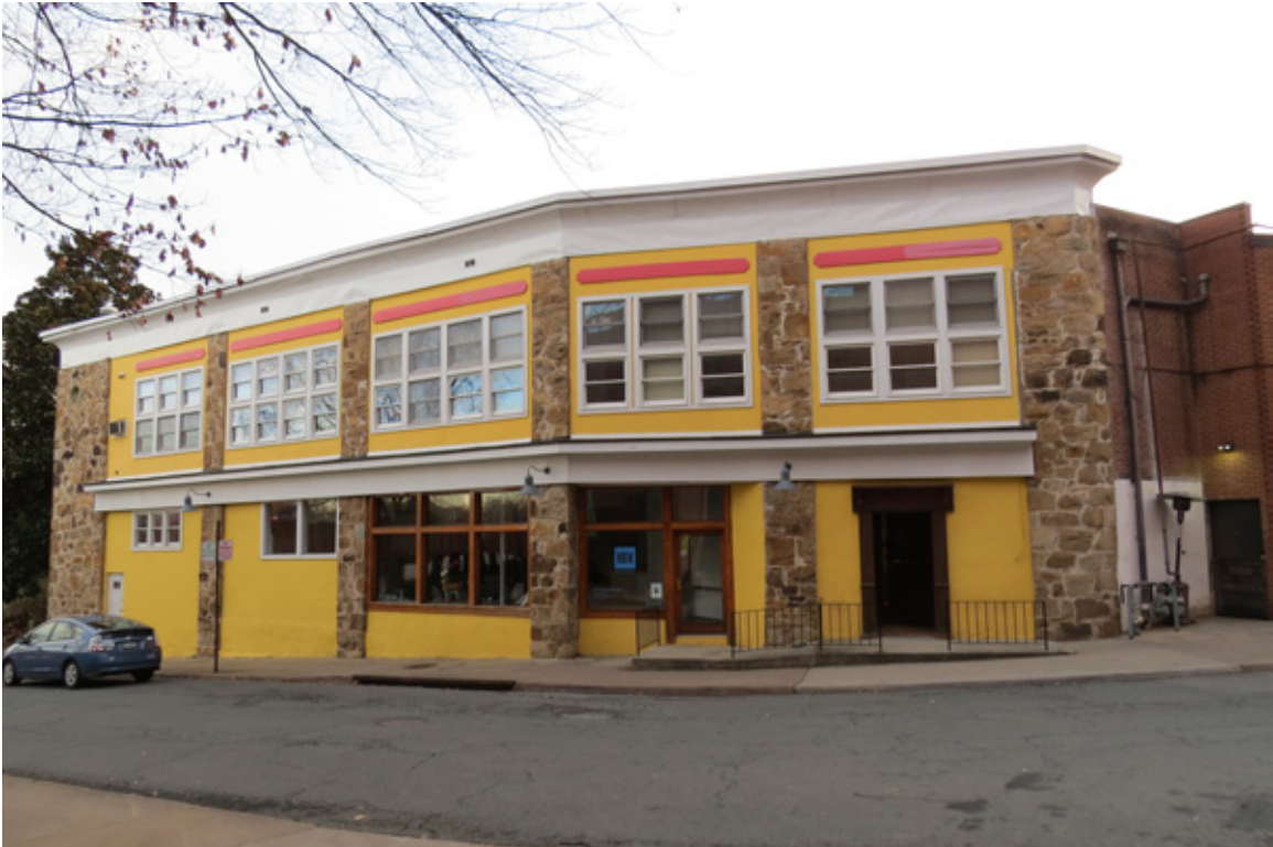
Adjacent structure at southwest corner
