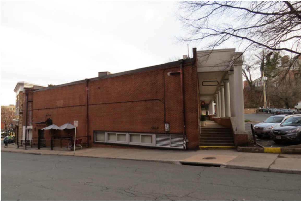
South façade, added after the original construction.
