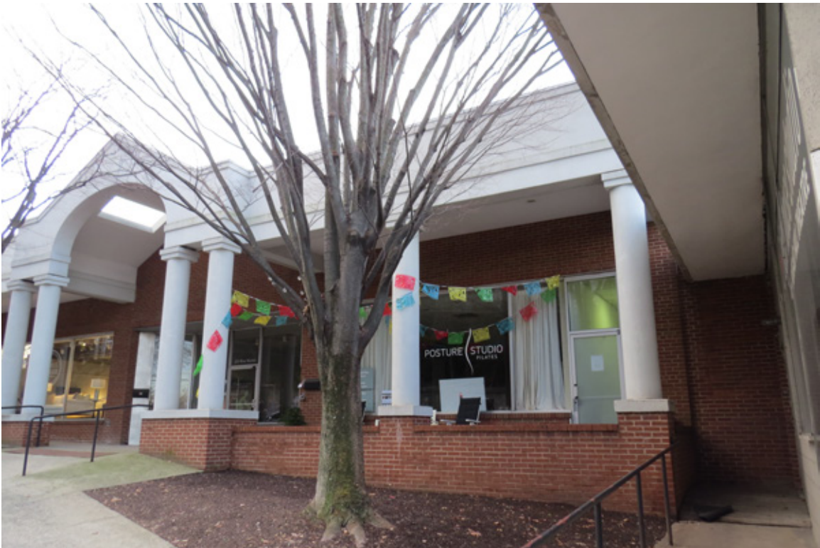
North façade detail, Vinegar Hill Theater to the right
