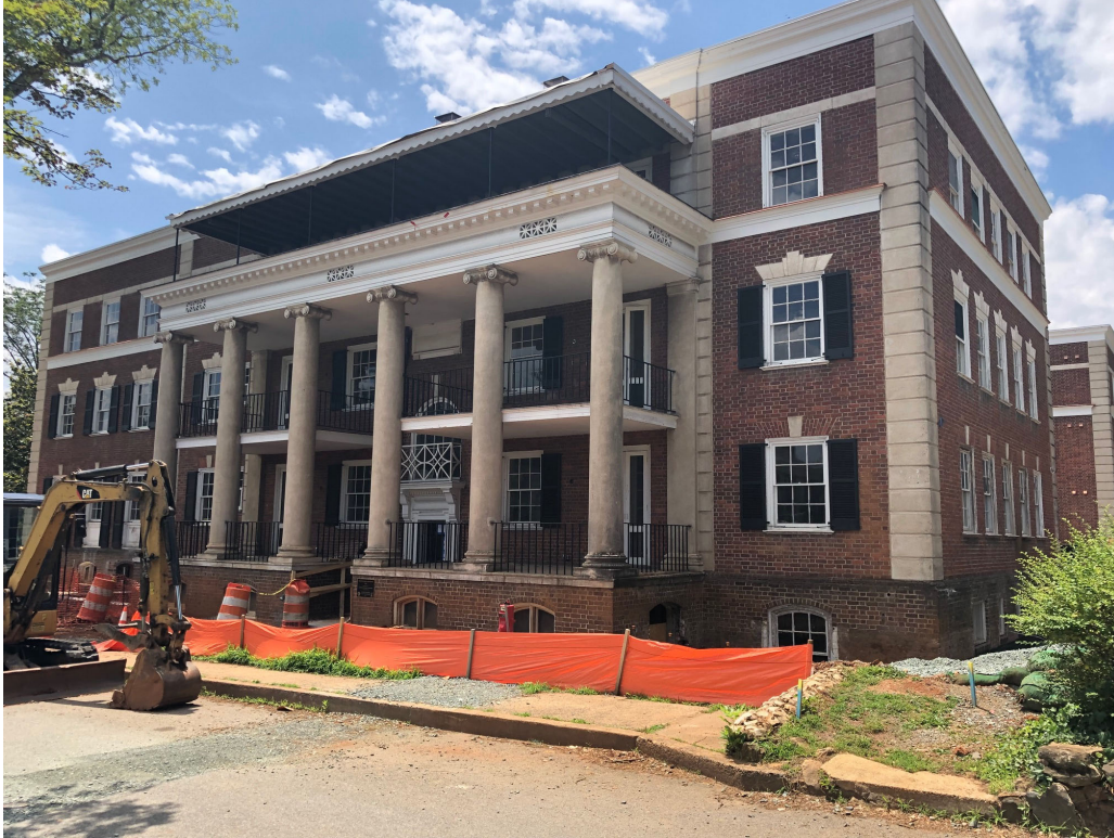
Preston Apartments – Currently under construction / renovation
