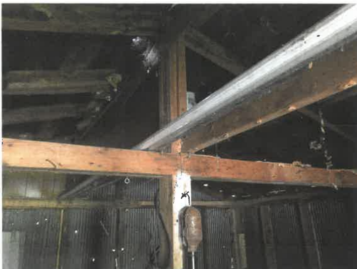
New shoring at existing ridge / roof structure
