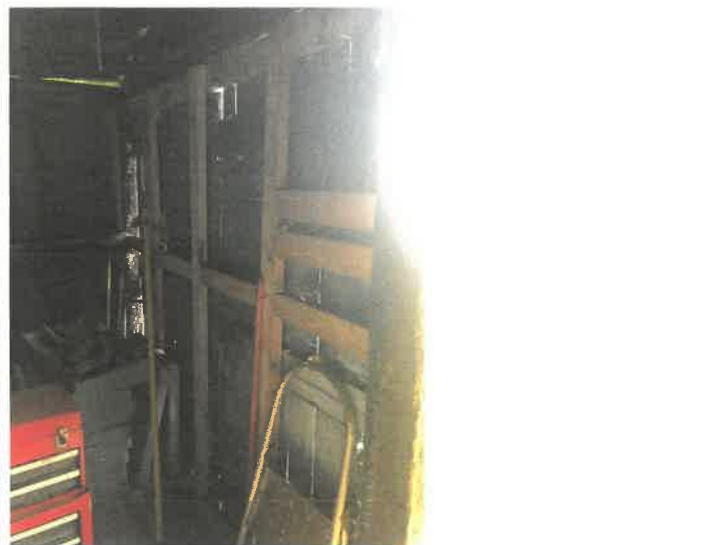
New reinforcement framing at exterior doors
