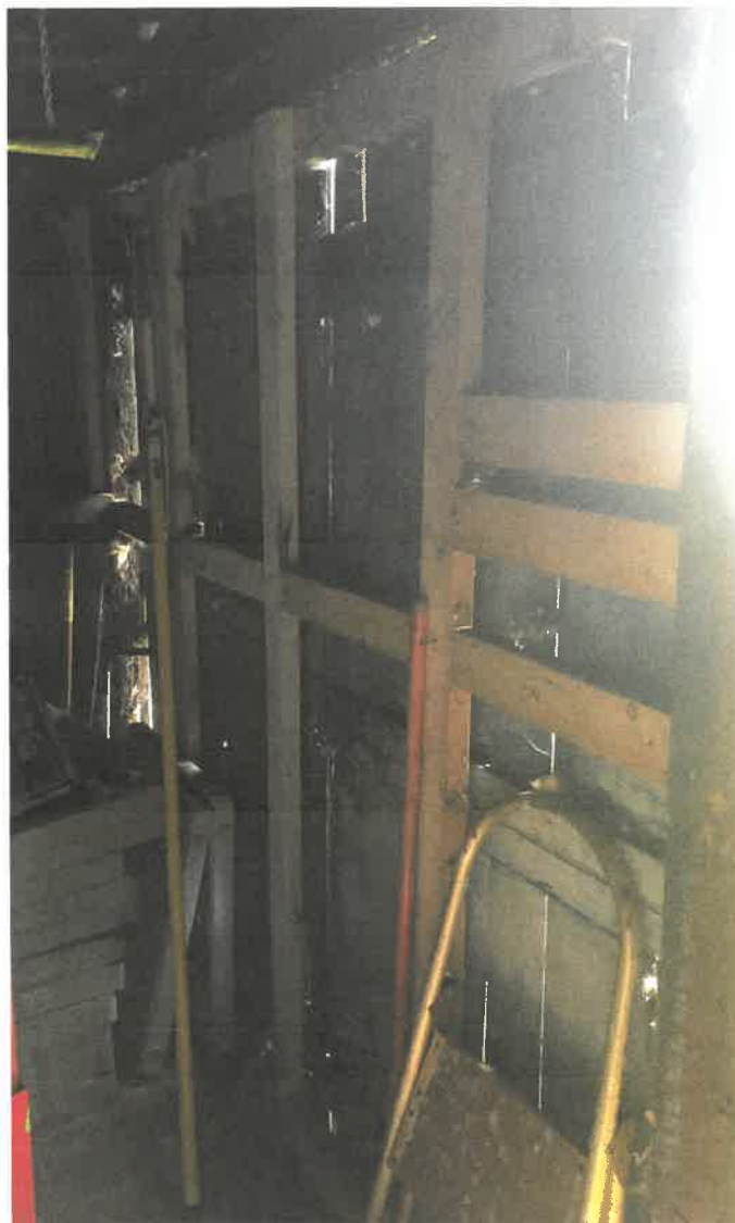
New supporting framing at existing doors.
