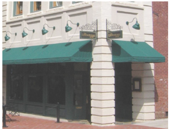
Gooseneck lights provide moderate levels of illumination and focus the light downward onto the awnings and the storefront.
