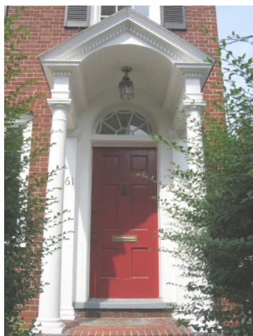
A pendant light fixture attached to the curved underside of this portico illuminates the entrance.
