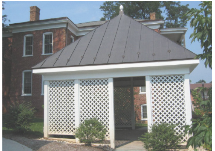
With diagonal lattice cladding and a hipped, standing-seam metal roof, this structure hides refuse containers from view.
