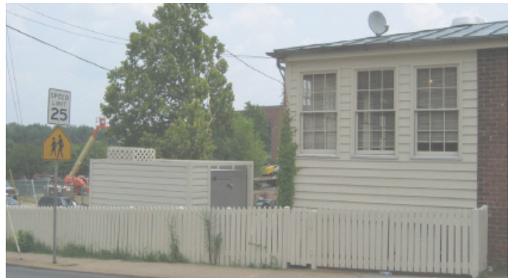
Mechanical equipment is placed to the rear of the building and screened with a material similar to that found on the site's primary structure.
