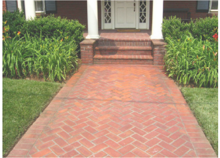
The use of brick laid in a herringbone pattern coordinates well with the dwelling's construction materials and traditional construction.
