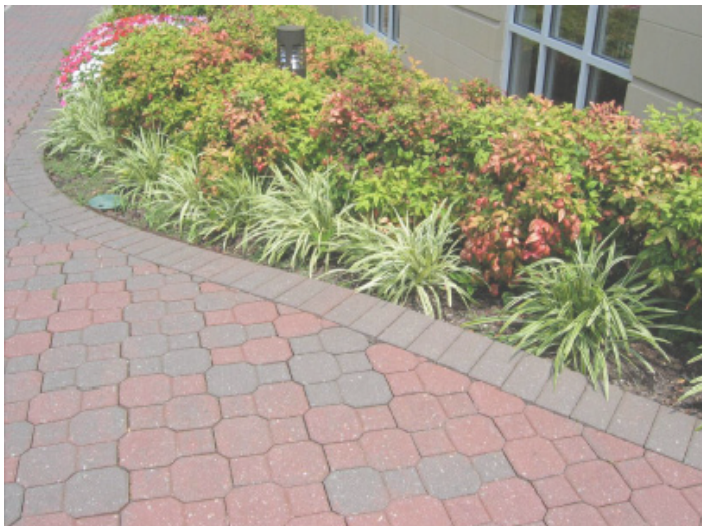
Interlocking concrete pavers laid in a traditional pattern may be appropriate for site walkways in historic district new construction.
