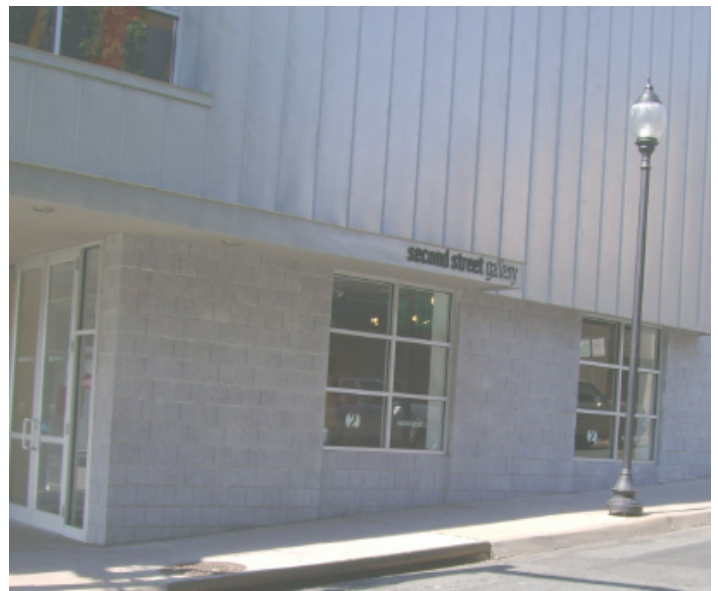
Concrete block differentiates the foundation of this building from the upper floors' metal cladding.
