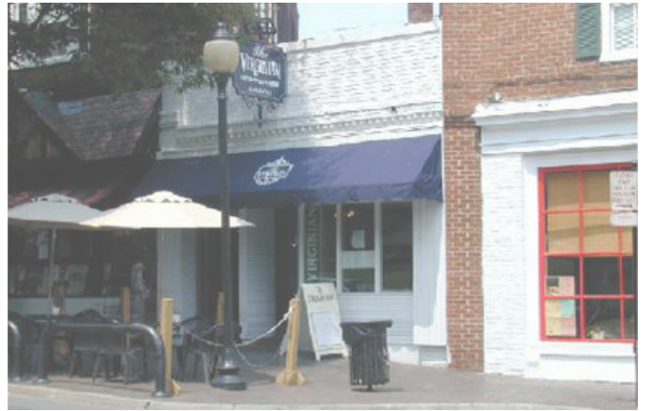
Historic commercial areas typically have adjoining structures and minimal spacing.
