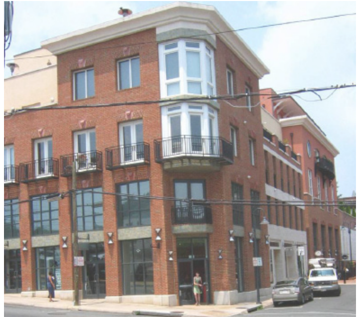
The massing of this new commercial building is varied due to its larger corner bay that wraps both sides before stepping down to three stories.
