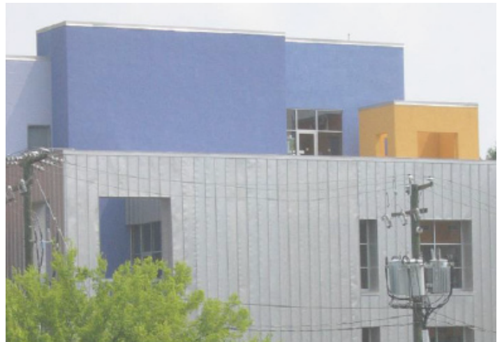
The bold use of color and geometric shapes to screen rooftop equipment from view becomes a design element in this example.
