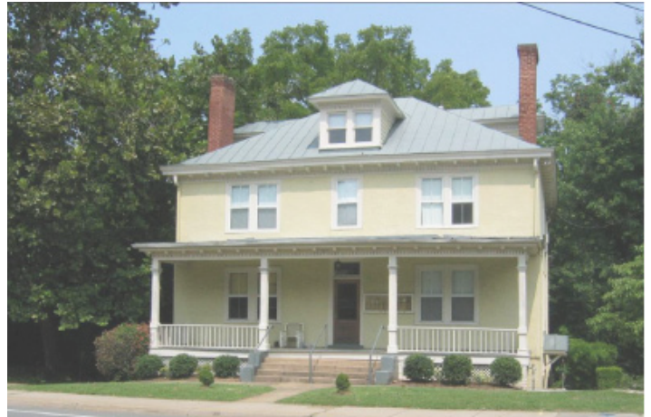
Standing-seam metal is a common roofing material in the historic districts as seen in this hipped roof example.
