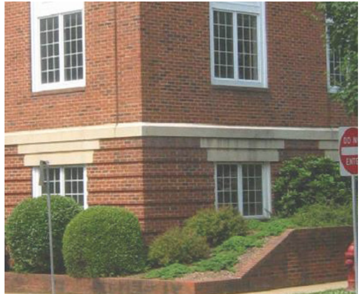
The rusticated brick foundation and cast water table and lintels reference traditional building styles found in this historic district.
