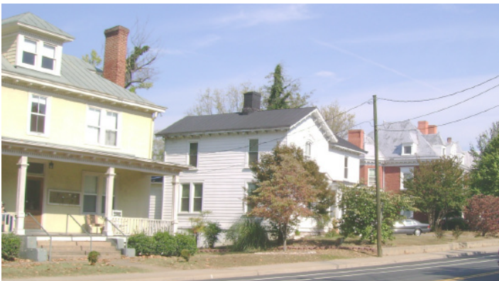
This row of turn-of-the-century residences illustrate the most common materials used in period construction: stucco, wood siding, and brick.
