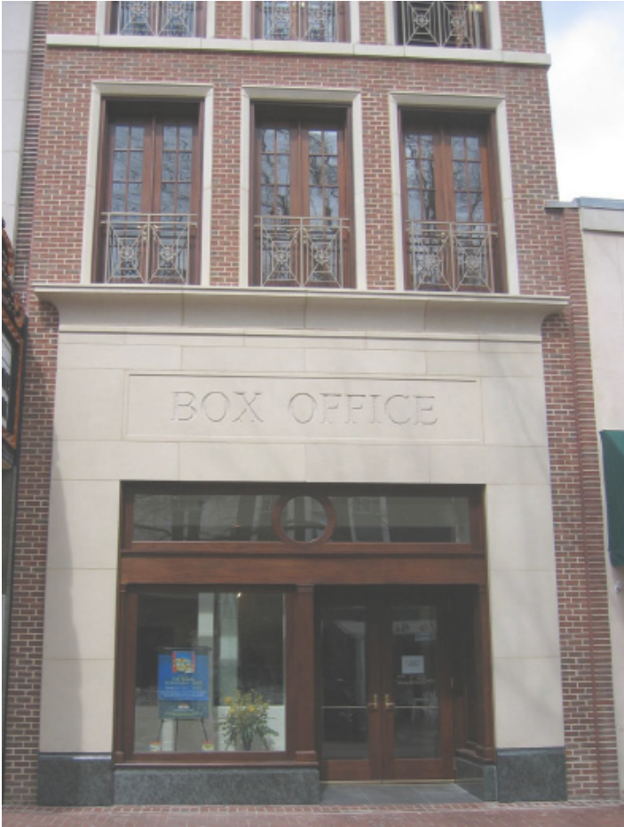
The use of varied materials on a commercial facade adds visual interest by dividing the building into different levels.
