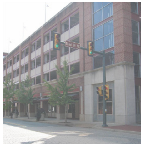
This parking garage facade uses bay divisions, storefronts, openings and changes in materials to help reduce its scale.
