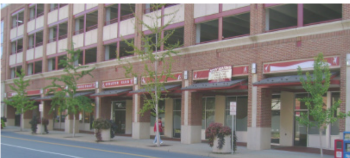
The first floor of this parking structure provides visual relief through the use of individual storefronts in recessed bays.
