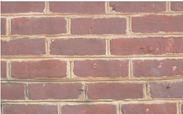
Lines struck in the mortar give bricks the appearance of a more uniform size and shape.
