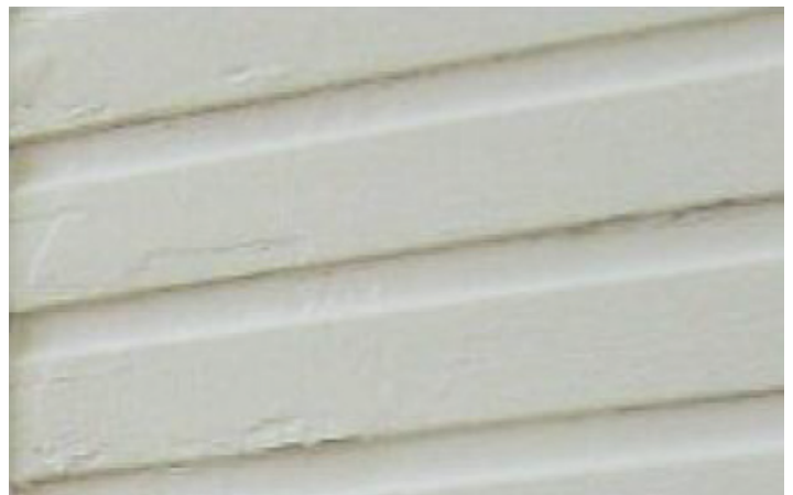
Shiplapped or novelty siding are the common terms for horizontal board siding with a simple detail as pictured above.
