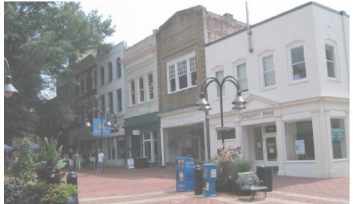
Most historic commercial buildings are designed with the traditional three-part facade.
