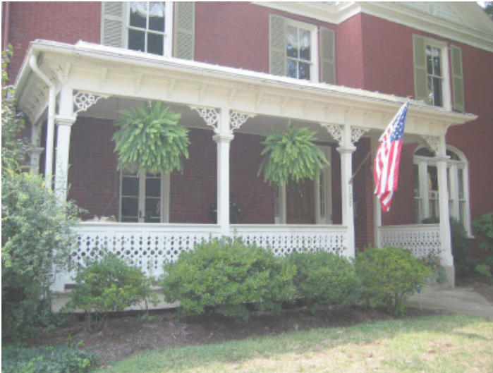
This well-preserved, one story, three bay porch features Italianate brackets at the roof-wall junction and lace-like scroll sawn corner brackets and balusters.
