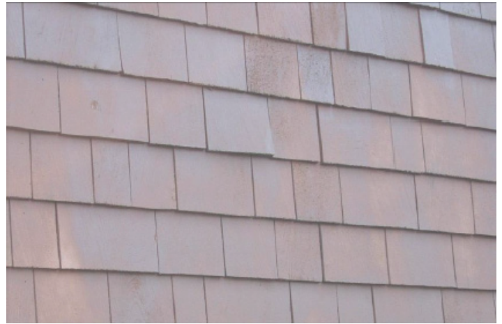
Wood shingles are often used as wall cladding in the Shingle, Craftsman, and Colonial Revival styles of architecture.
