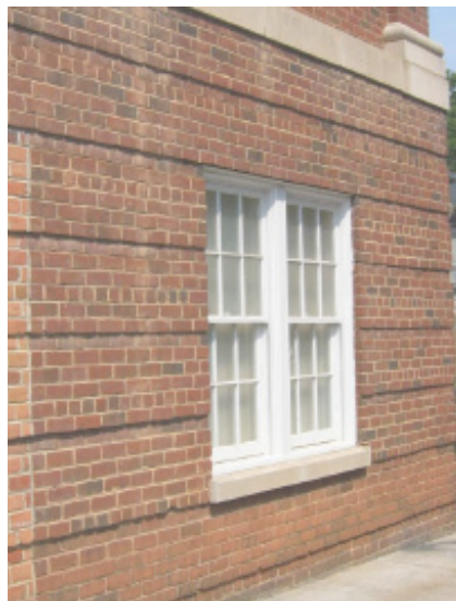
Stringcourses add strength to the appearance of this brick foundation.
