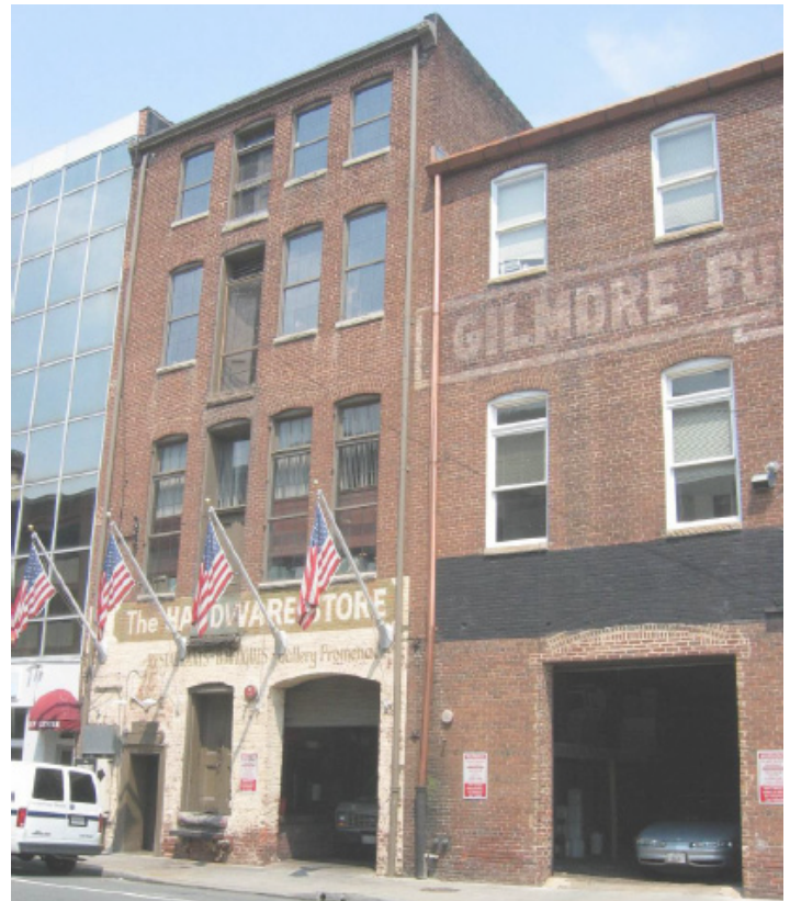
Historic openings on the rear of these downtown buildings have been modified for automobile access while retaining the integrity of the secondary facades.
