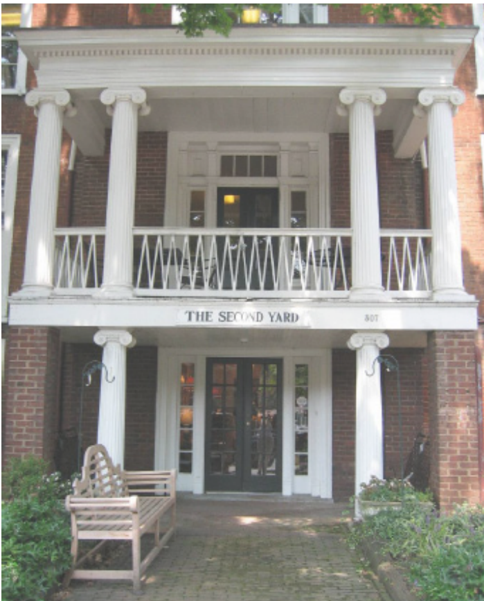
This two-story porch in the Greek Revival style uses Ionic columns capped by a simple classical entablature.
