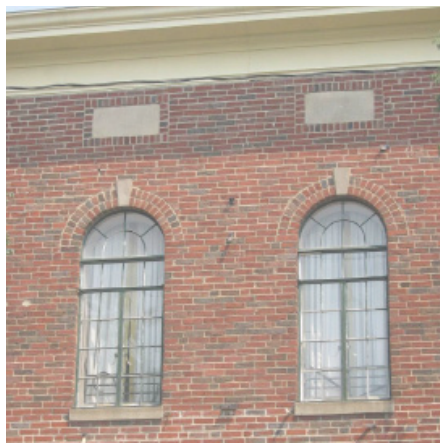
Metal casement with semi-circular brick arches and keystones.
