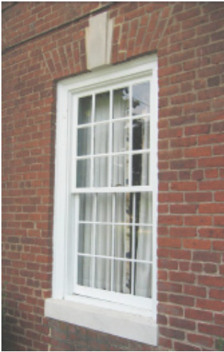
Twelve-over-twelve with keystone and brick flat arch.
