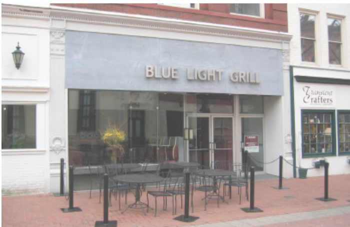
This contemporary storefront is framed by the building's original, architecturally significant cornice and pilasters.
