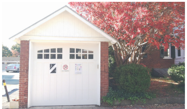
“The Garage,” an arts and music venue, retains the character of a residential garage from the exterior but has been retrofitted to accommodate public shows.
