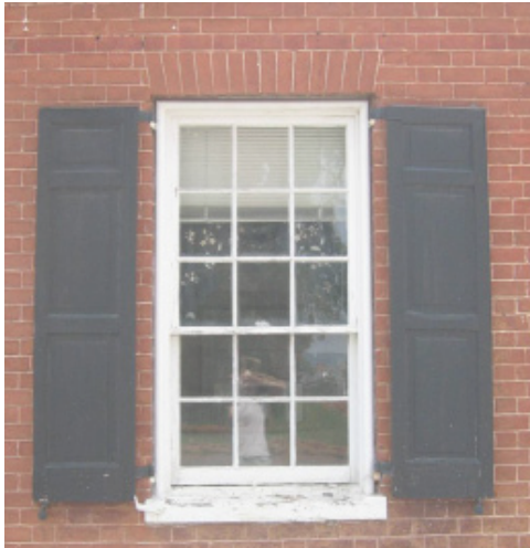
Nine-over-six with operable shutters and jack arch.
