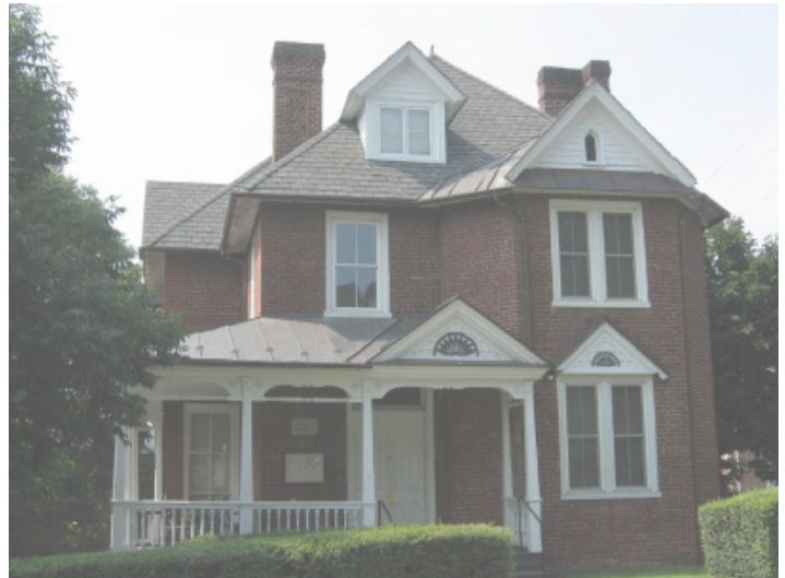
d. Complex Roof
