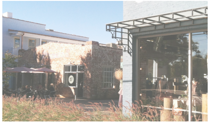
A series of garage spaces on West Main Street were rehabilitated into shops and restaurants.
