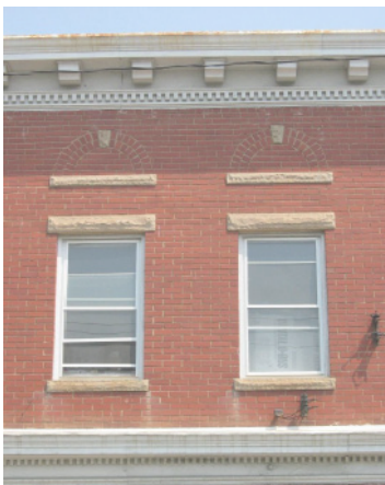
One-over-one with rough faced stone lintel.
