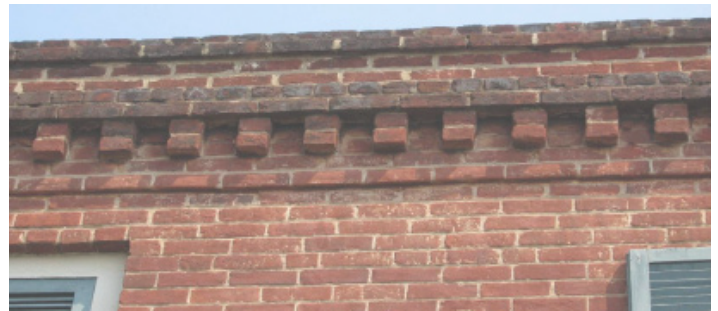
Decorative brickwork forms a classical cornice with dentils.
