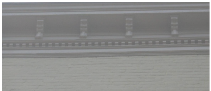
This Italianate cornice uses brackets to support the overhanging eave.
