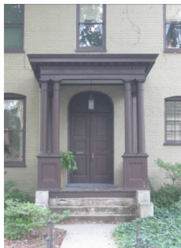
Paired columns rest on pedestals and support a classical entablature framing the double-entry doors capped by a fanlight.
