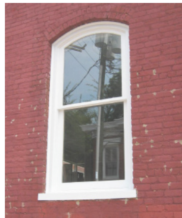
One-over-one with segmental brick arch.
