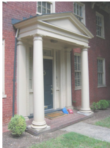
A six panel door with transom and sidelights flanked by pilasters is the central feature of this classical entrance feature with pediment and columns.
