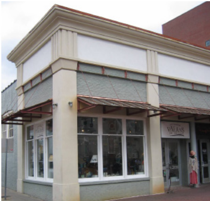
These metal fixed canopies blend in well with this contemporary storefront design.
