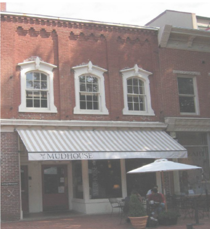
A modern awning with no fabric on the sides can be an alternative to more traditional designs.
