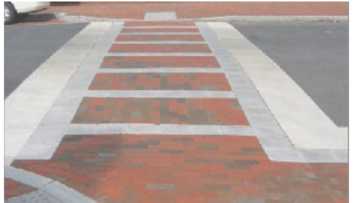
Brick crosswalks with granite details highlight pedestrian crossings in the area surrounding the Albemarle County Courthouse.
