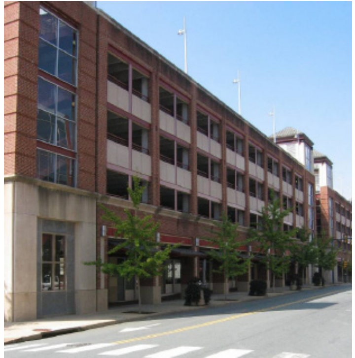
Uniform bays, stair towers, recessed storefronts with awnings and street trees add interest to this large, municipal facility.
