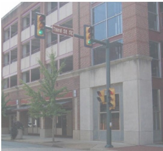
Traditional mast-arm traffic signals fit the scale of this intersection.
