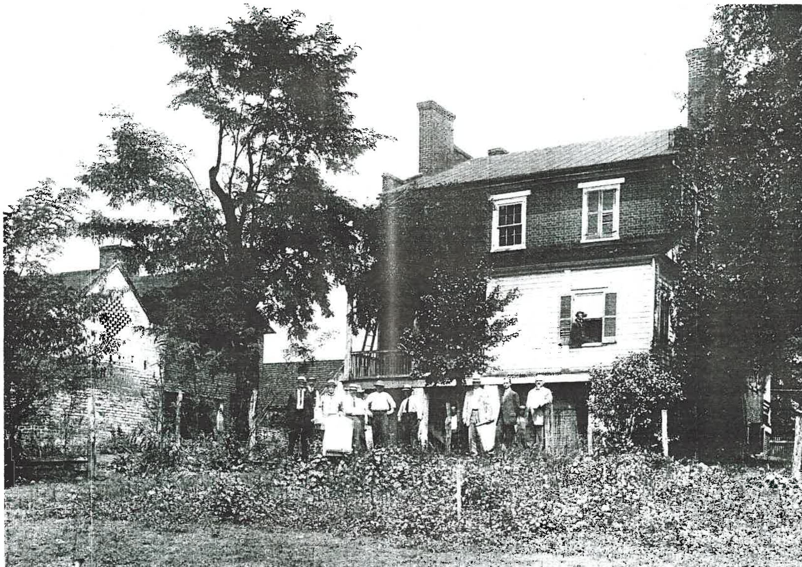
The individuals, reading left to right, are: R. F. Webb, a high school teacher; Supt. James G. Johnson; J. E. Harrison of the Charlottesville Lumber Co., contractors; Charles E. Chisholm, a foreman for excavation, etc.; Robert E. Carter, in charge of construction; Dr. J. E. Early, W. C. Scott, and A. Russow, school board building committee. In 1871 school No. 4 was taught in small brick building at left.
