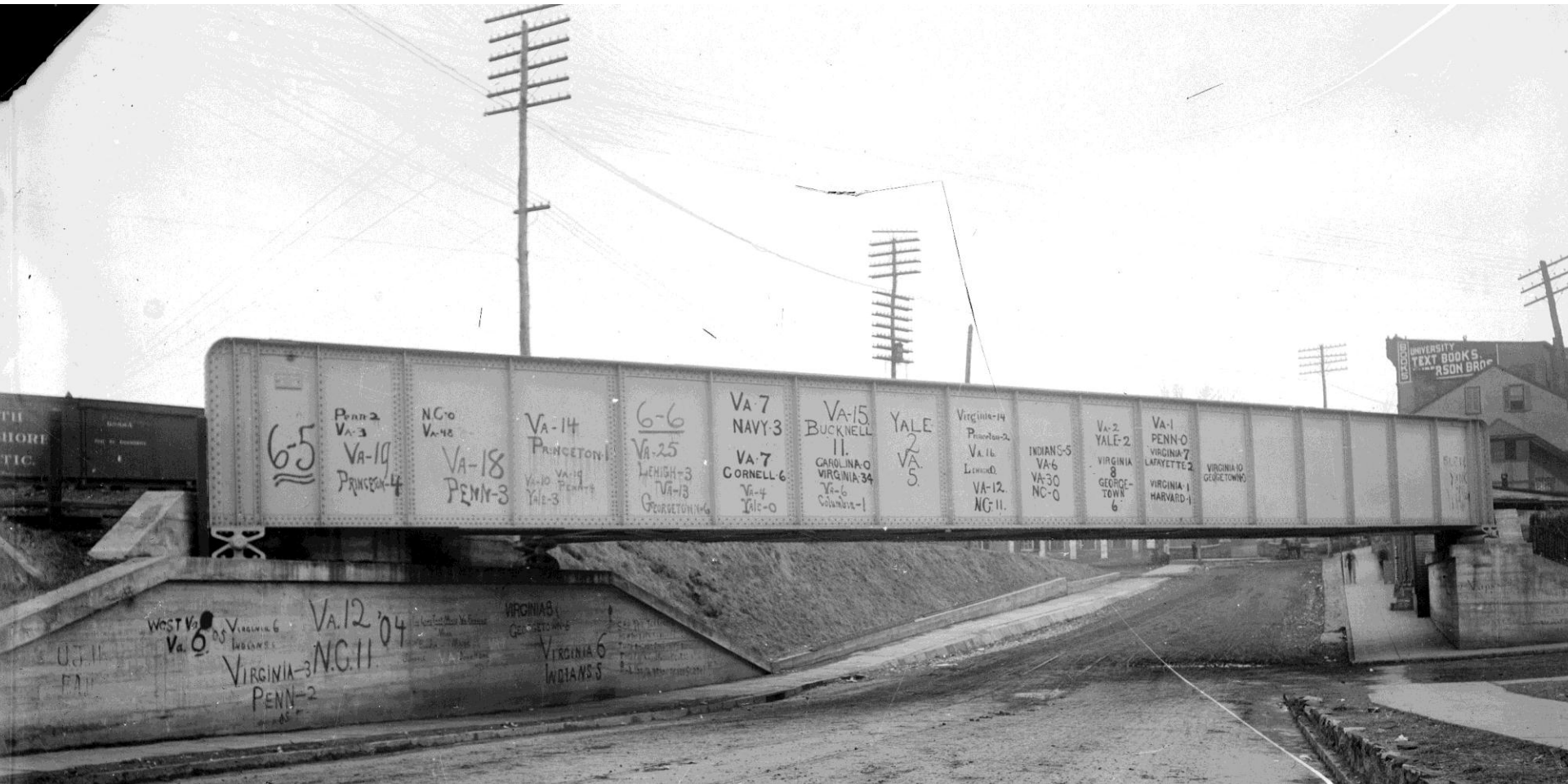
THE C&O RAILROAD "BRIDGE OF SCORES"
