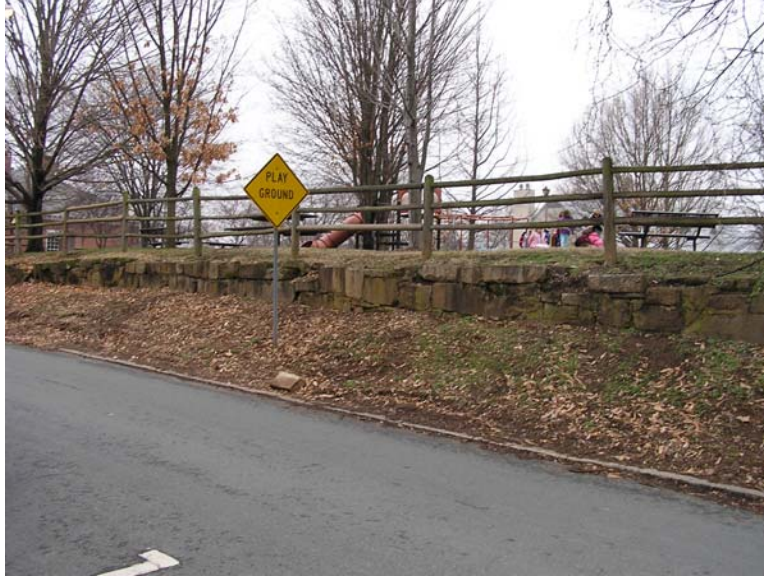
McGuffey Park showing stone retaining wall
