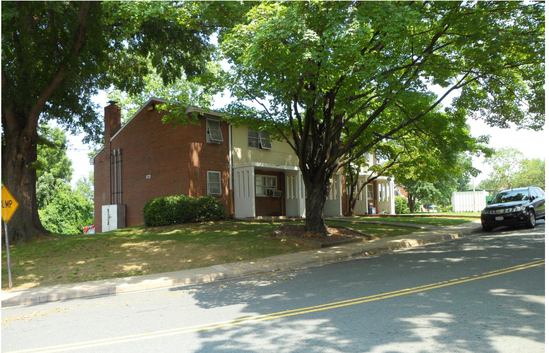
View of two units (four bedroom on the left and five bedroom on the right) on the north side of Hardy Drive) Photo by Kristin Rourke
