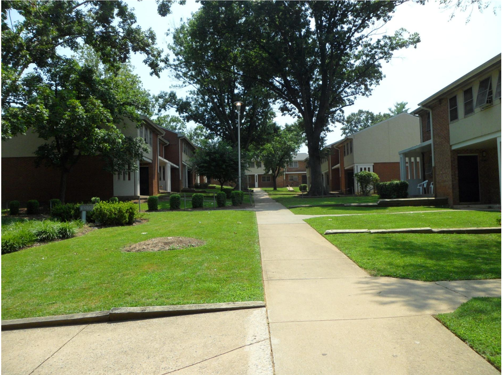
View of one row of 2 and 3 Bedroom Units south of Hardy Drive. Photo by Kristin Rourke
