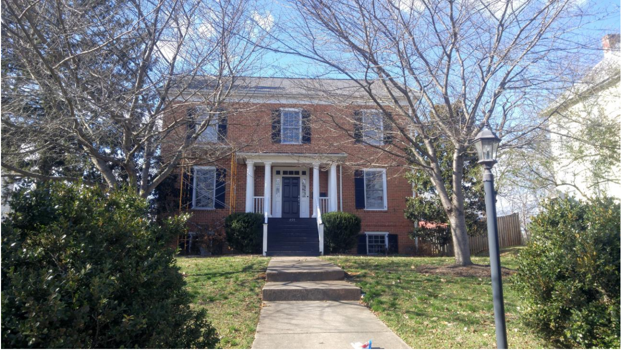
Figure 3: East elevation of subject building.
