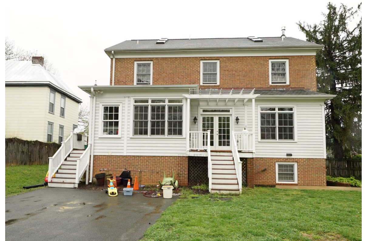
EXISTING BACK PORCH
