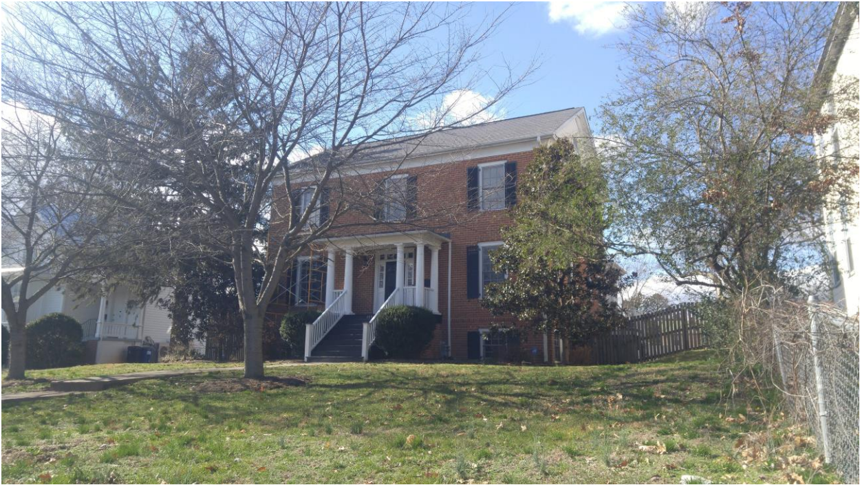
Figure 4: Oblique view, facing southwest, of subject building.
