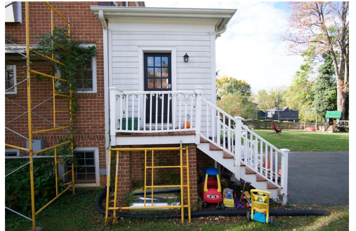
EXISTING NORTH ENTRY
