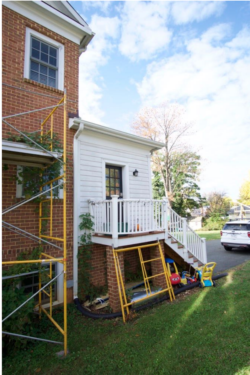
EXISTING NORTH ENTRY
