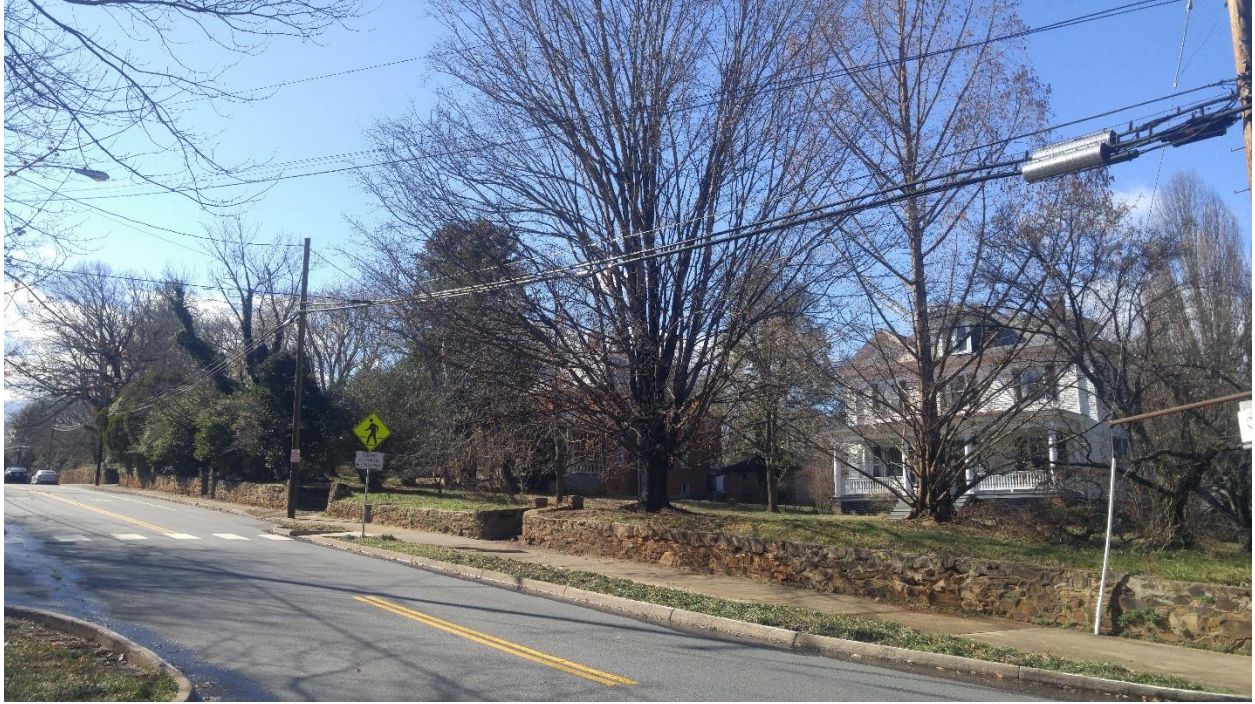
Figure 3: Oblique view, facing southwest, of subject building in context of district. 751 Park Street at right.
