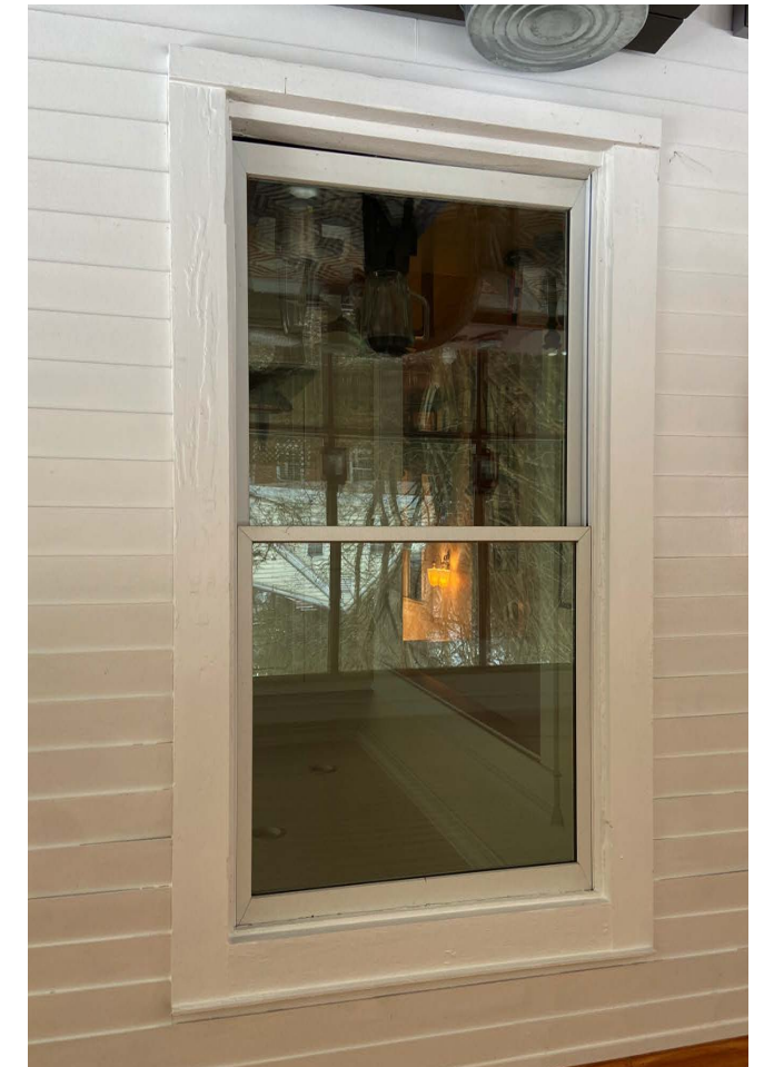
EXISTING WINDOW & FIBER CEMENT LAP SIDING ON WEST PORCH
