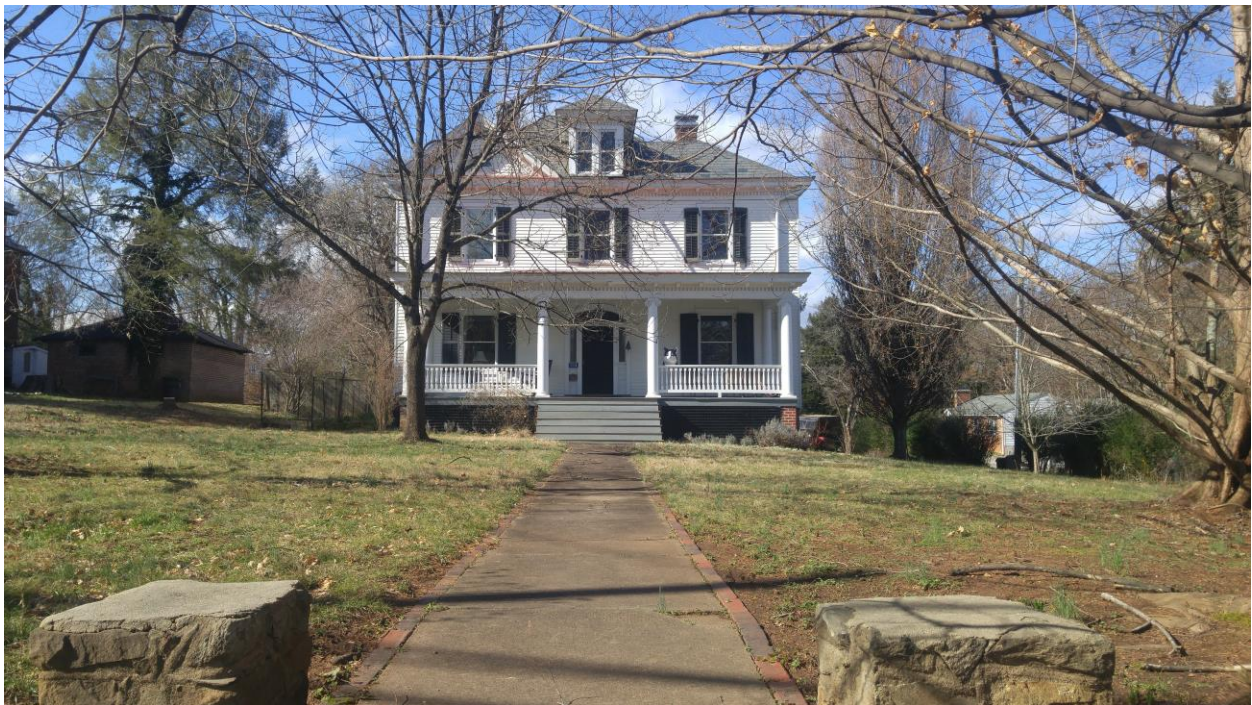
Figure 2: East elevation of subject building.
