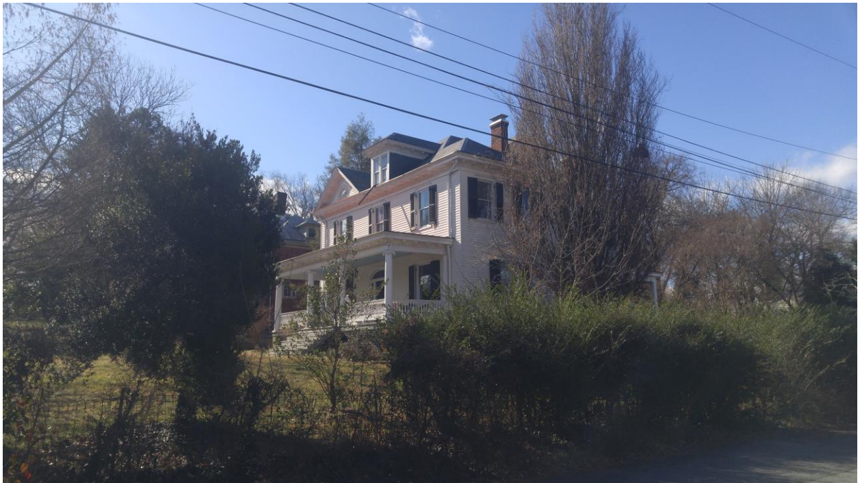
Figure 4: Oblique view, facing southwest, of subject building.
