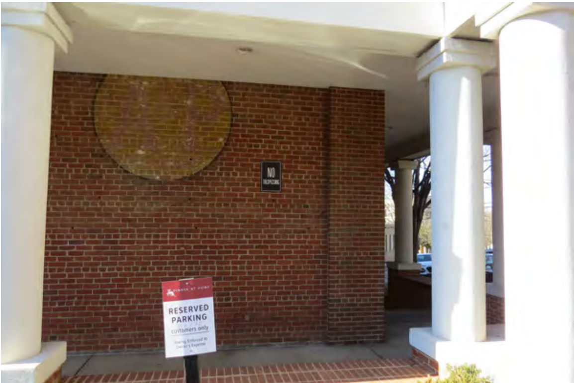
Northeast corner of the building: brickwork from three different periods of construction
