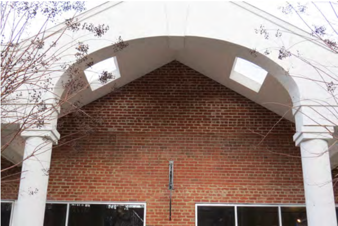
Added brickwork in portico of east façade
