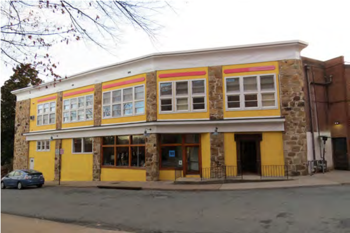
Adjacent structure at southwest corner
