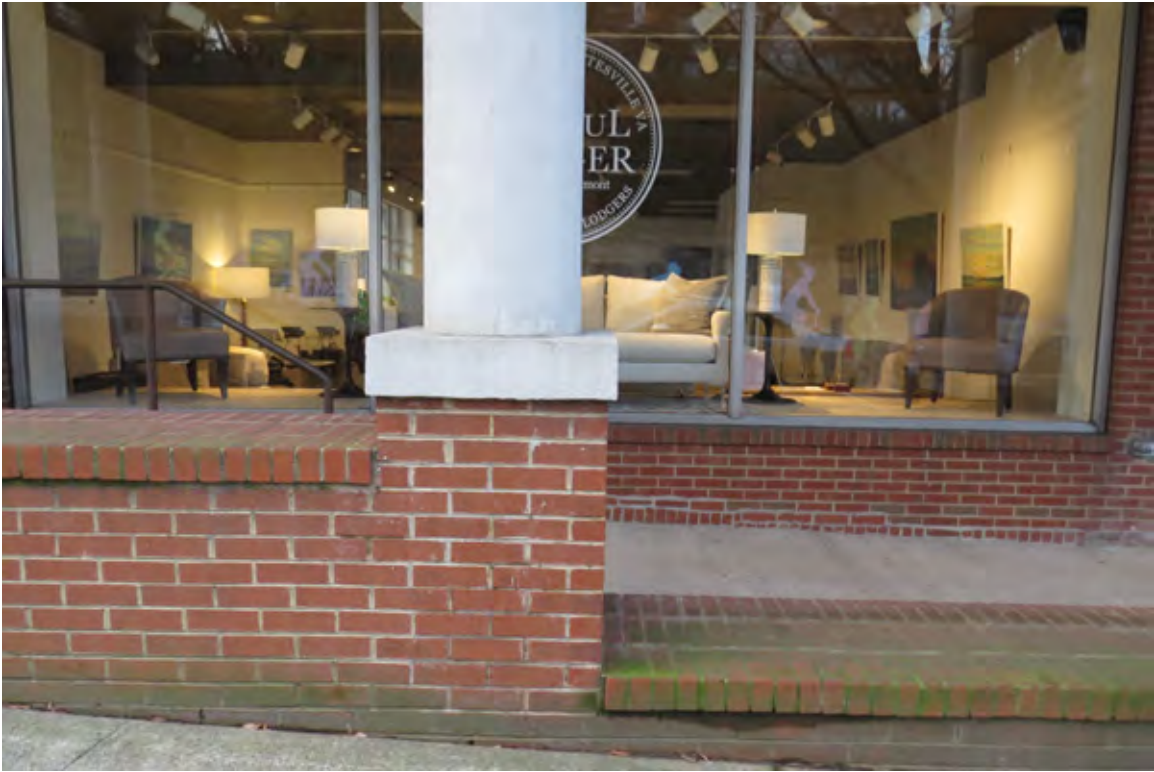
North façade detail: brickwork from three different periods of construction
