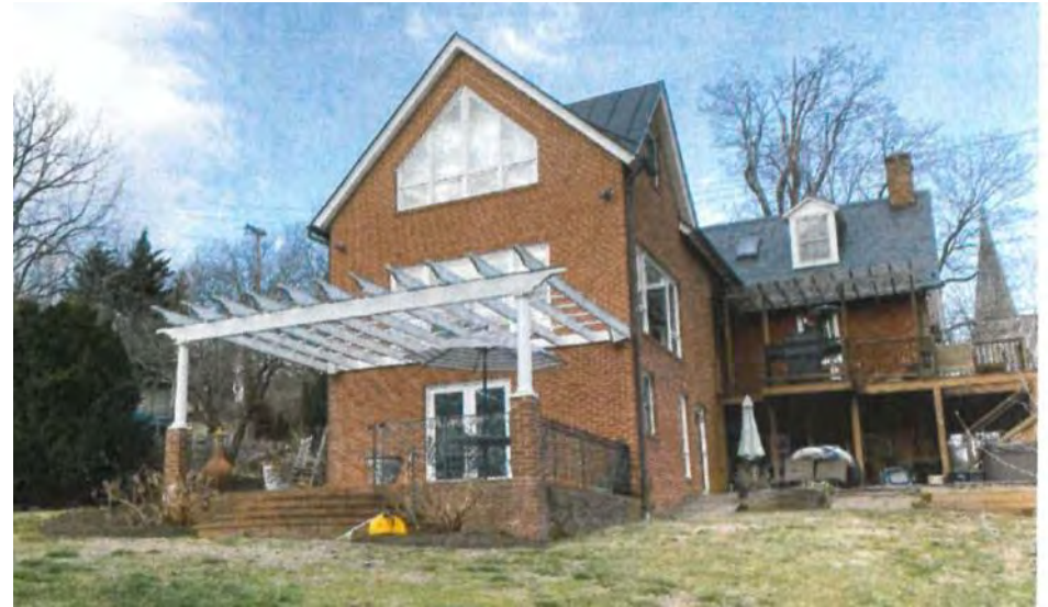
Existing - Northeast Elevation (from river)
