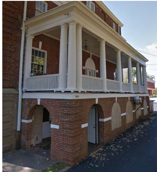
Figure 2: Filled-in arched basement openings at 165 Rugby Road
