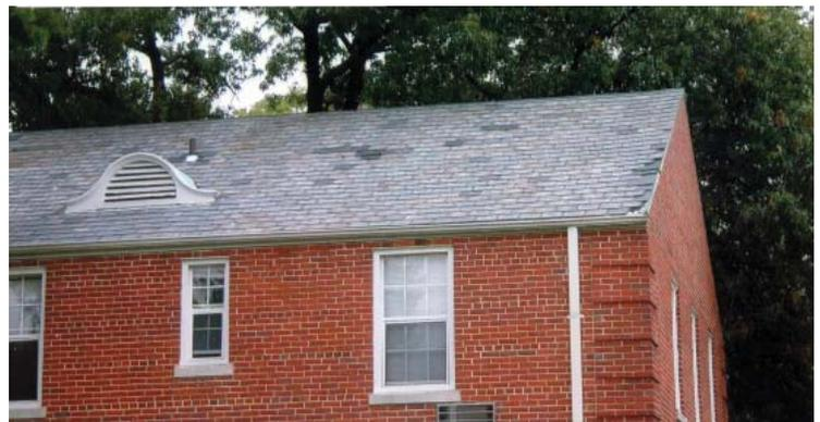
*Close up of damaged and previously repaired slate.*
