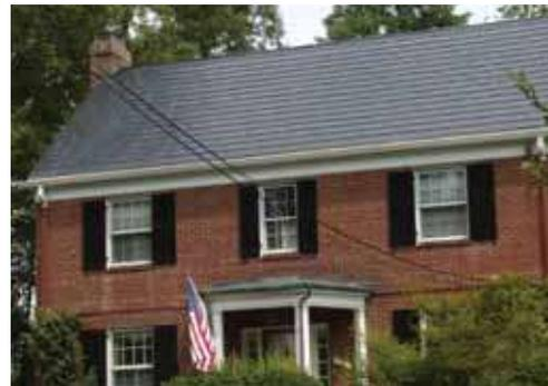
**Not Recommended:** [87] Historic roofing materials in good condition should be retained rather than replaced with another material perceived as more sustainable, such as, in this case, solar roofing shingles.
