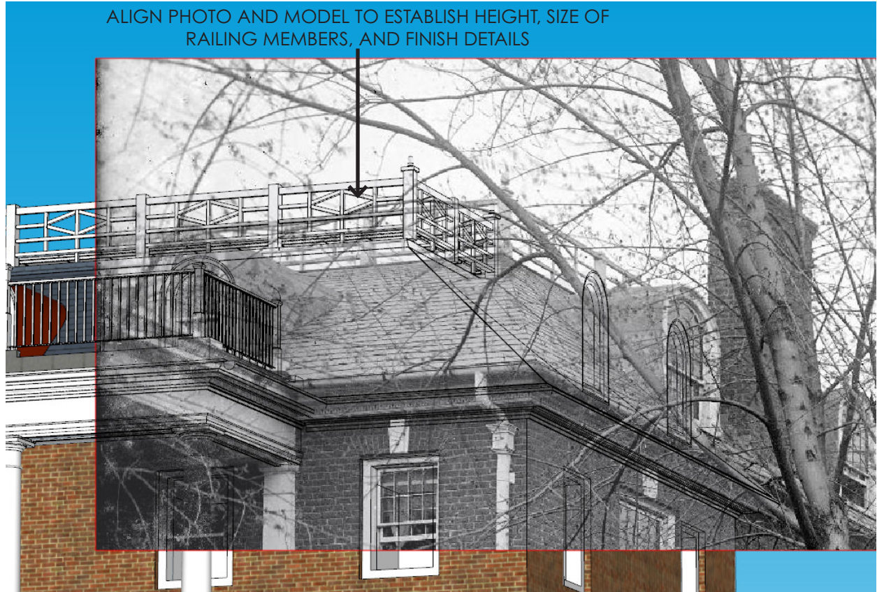
STEP 4: RECREATING THE HISTORIC RAILING THROUGH A "PHOTOMATCH" PROCESS, ALIGNING PERSPECTIVES DIGITALLY
