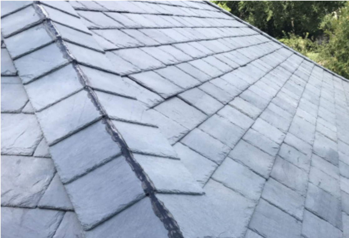
HIP DETAIL (BELLAFORTE SLATE)
