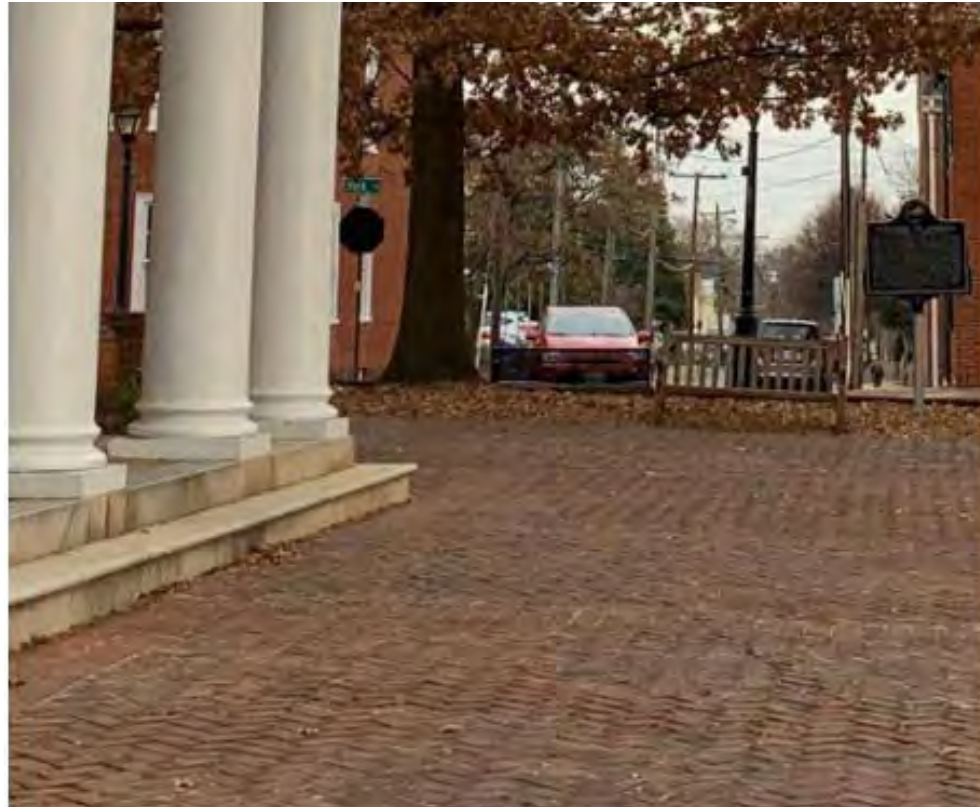
PAVING AT SITE, 1803 PLAZA
