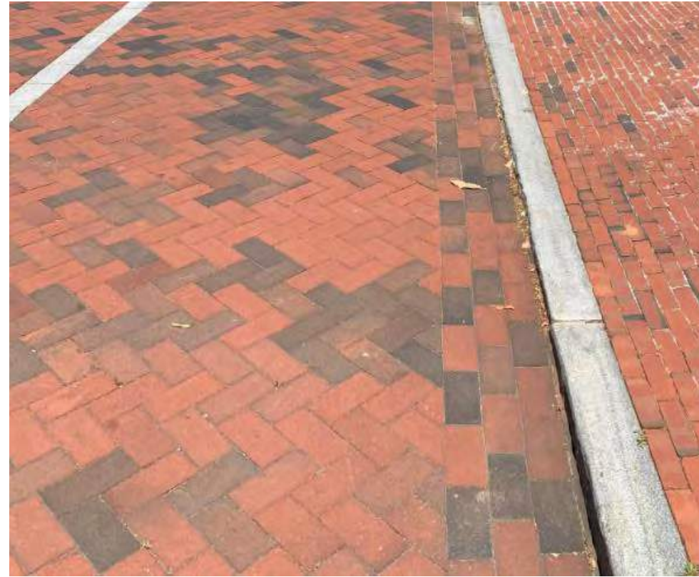
PAVING AT SITE, PARK STREET
