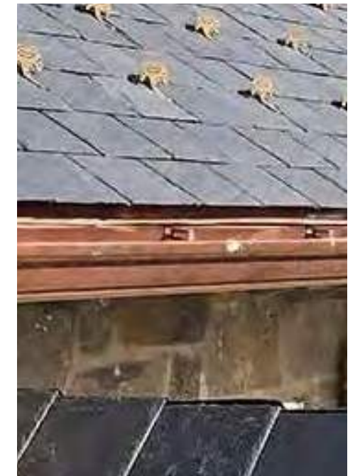
SLATE ROOFING AND COPPER GUTTER
