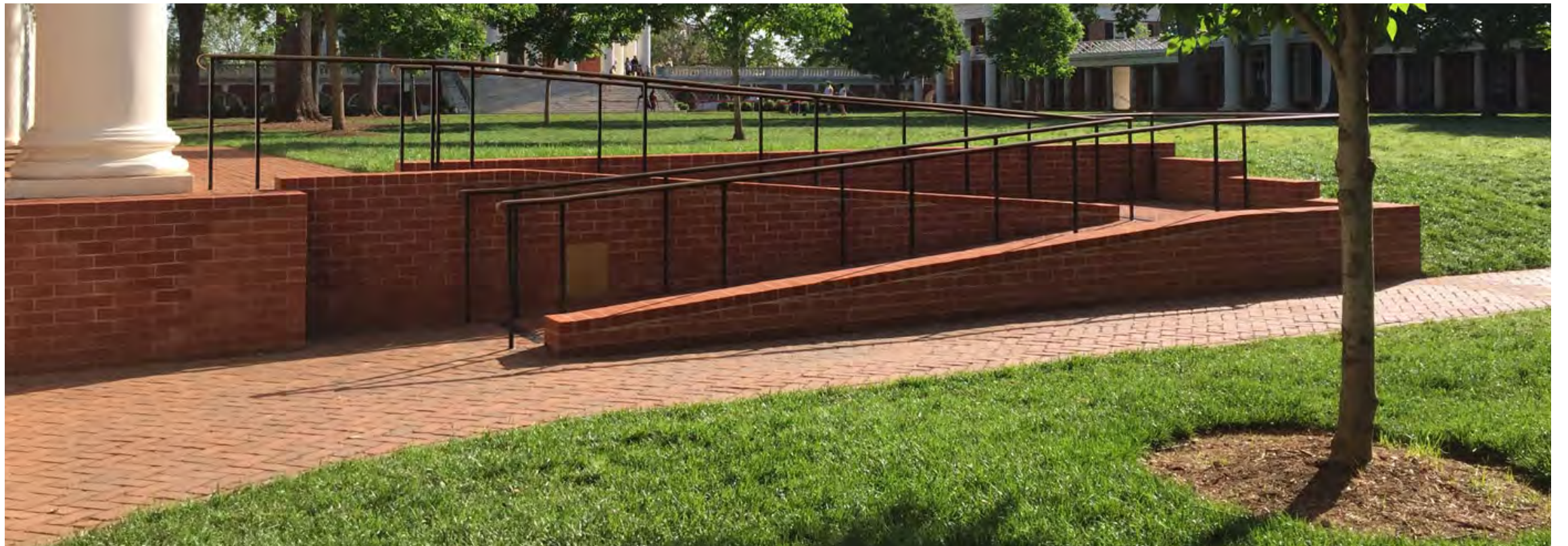
BRICK RAMP AND ORNAMENTAL METAL HANDRAIL
