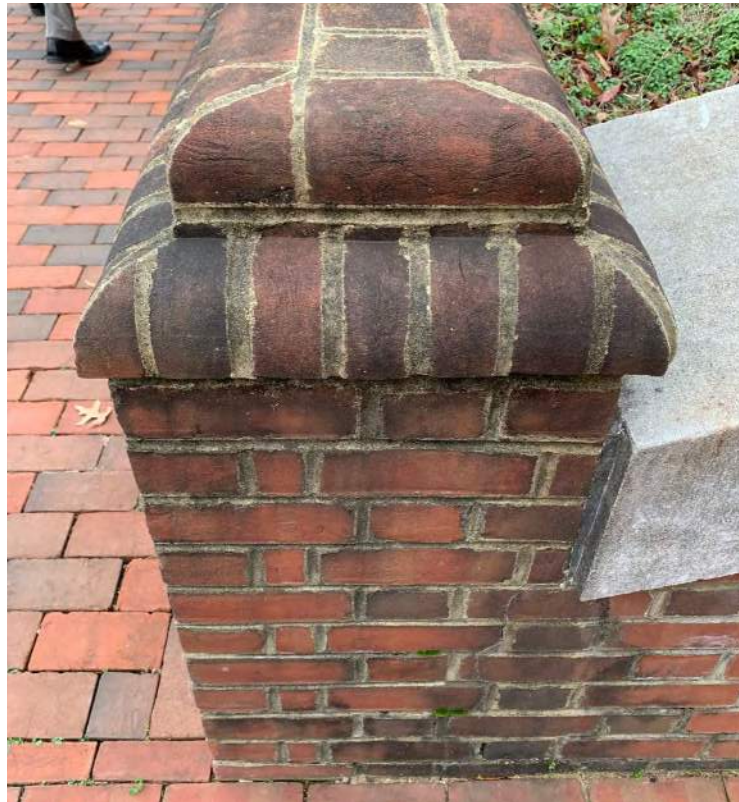
BRICK WALL - WEST SITE PRECEDENT
