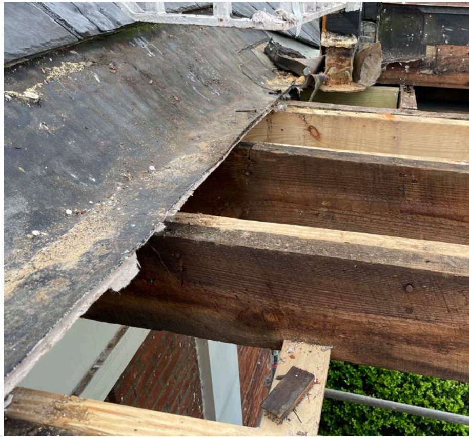
AUGUST 2022 - DESIGN DEVELOP, IN PARTNERSHIP WITH DUNBAR STRUCTURAL ENGINEERING, PROVIDED A DESIGN TO STABILIZE, REINFORCE AND ENSURE THE LONGEVITY OF THE HISTORIC FRAMING, WHILE STRENGTHENING THE FAILING RAILING CONNECTIONS. EVALUATION OF THE HISTORIC COLUMNS WAS PERFORMED, AND THE FRONT PORCH BEAM WAS REINFORCED.
