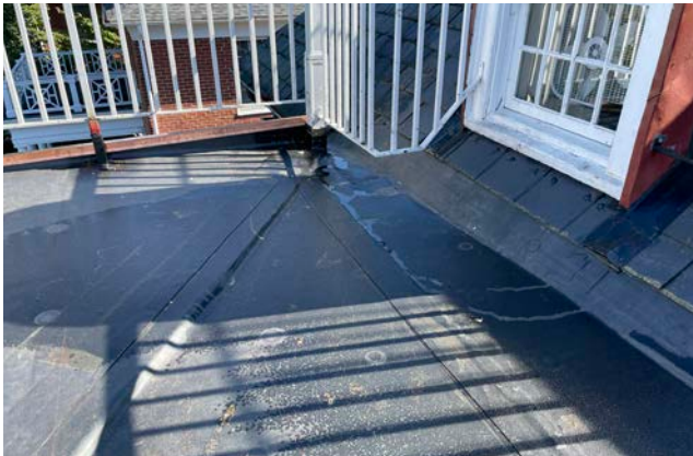
SEPTEMBER 2022 - NEW EPDM RUBBER ROOFING MEMBRANE OVER PITCHED RIGID INSULATION INSTALLED, NEW PITCH POCKETS / WATERPROOFING BOOTS INSTALLED AT RAILING POSTS.
