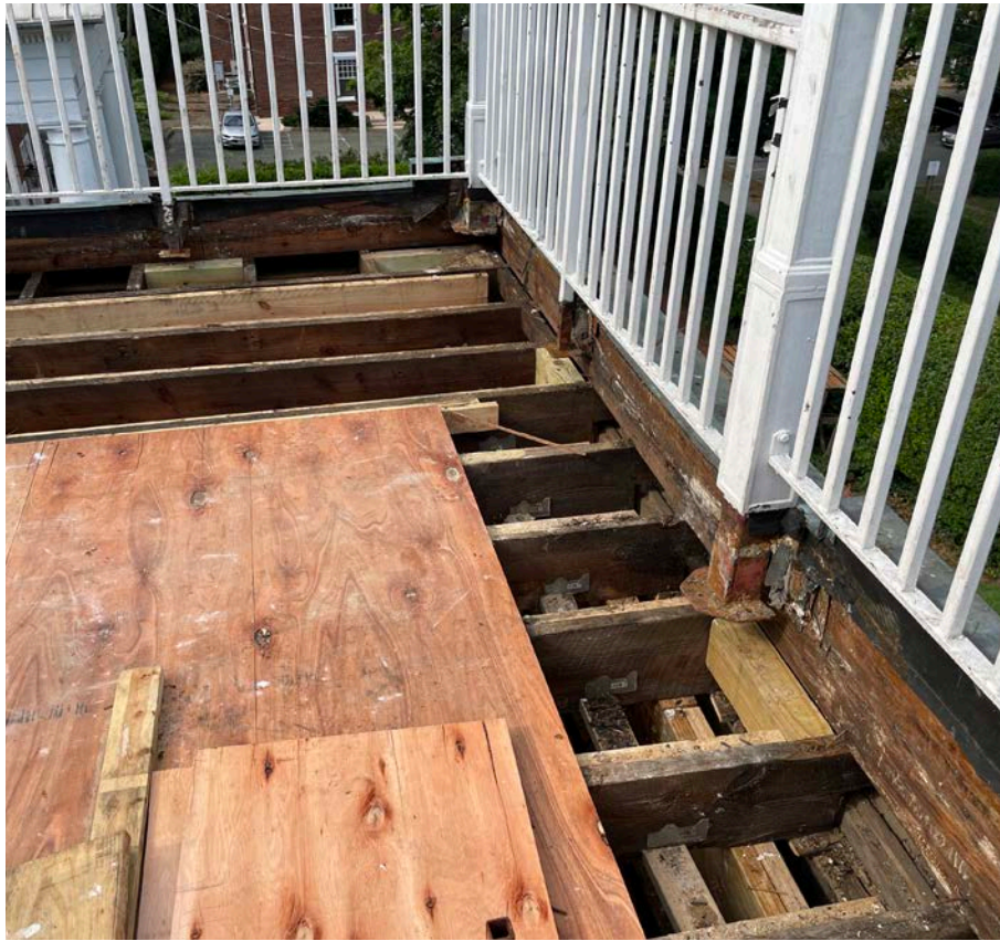
AUGUST 2022 - DESIGN DEVELOP, IN PARTNERSHIP WITH DUNBAR STRUCTURAL ENGINEERING, PROVIDED A DESIGN TO STABILIZE, REINFORCE AND ENSURE THE LONGEVITY OF THE HISTORIC FRAMING, WHILE STRENGTHENING THE FAILING RAILING CONNECTIONS. EVALUATION OF THE HISTORIC COLUMNS WAS PERFORMED, AND THE FRONT PORCH BEAM WAS REINFORCED.
