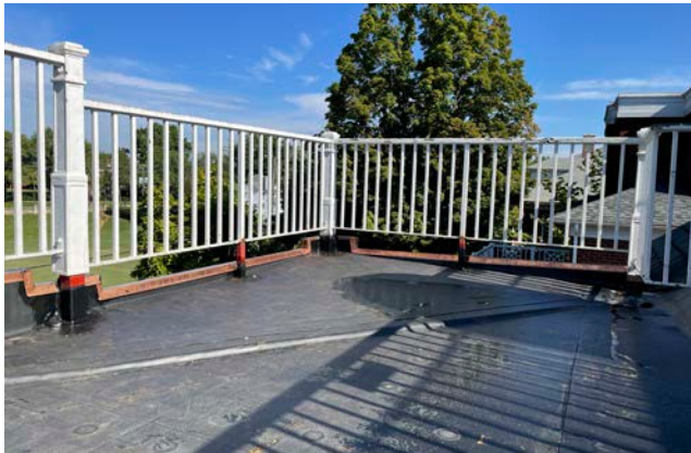
SEPTEMBER 2022 - NEW EPDM RUBBER ROOFING MEMBRANE OVER PITCHED RIGID INSULATION INSTALLED, NEW PITCH POCKETS / WATERPROOFING BOOTS INSTALLED AT RAILING POSTS.
