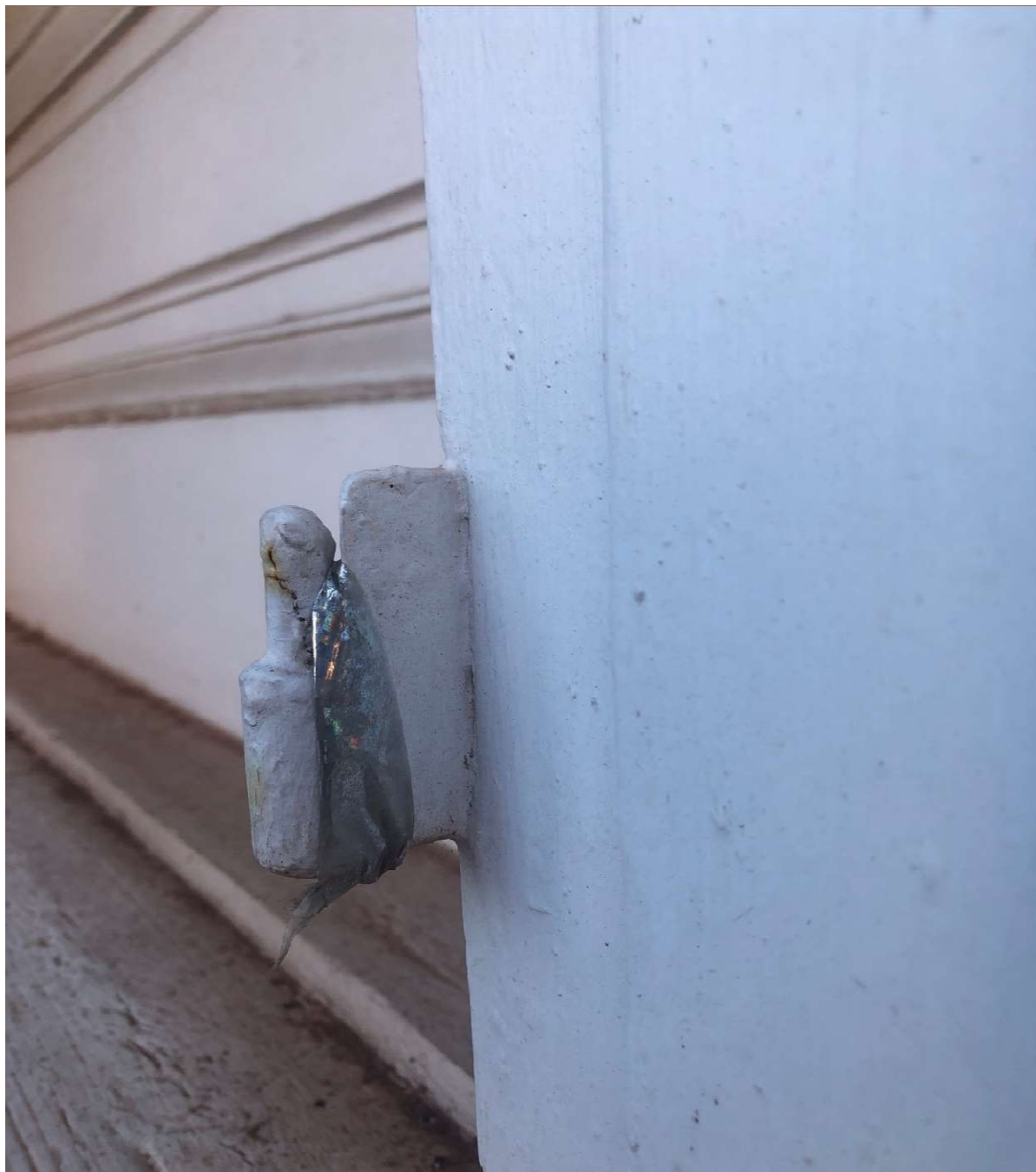
PHOTO 12 B – ORIGINAL SHUTTER PINS
