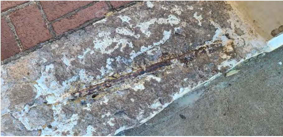
FRONT PORTICO - DETERIORATION TO PRECAST EXPOSING REINFORCING
