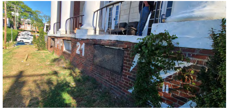
FRONT PORTICO - BRICK DETERIORATION PLYWOOD INFILLS TO WINDOWS
