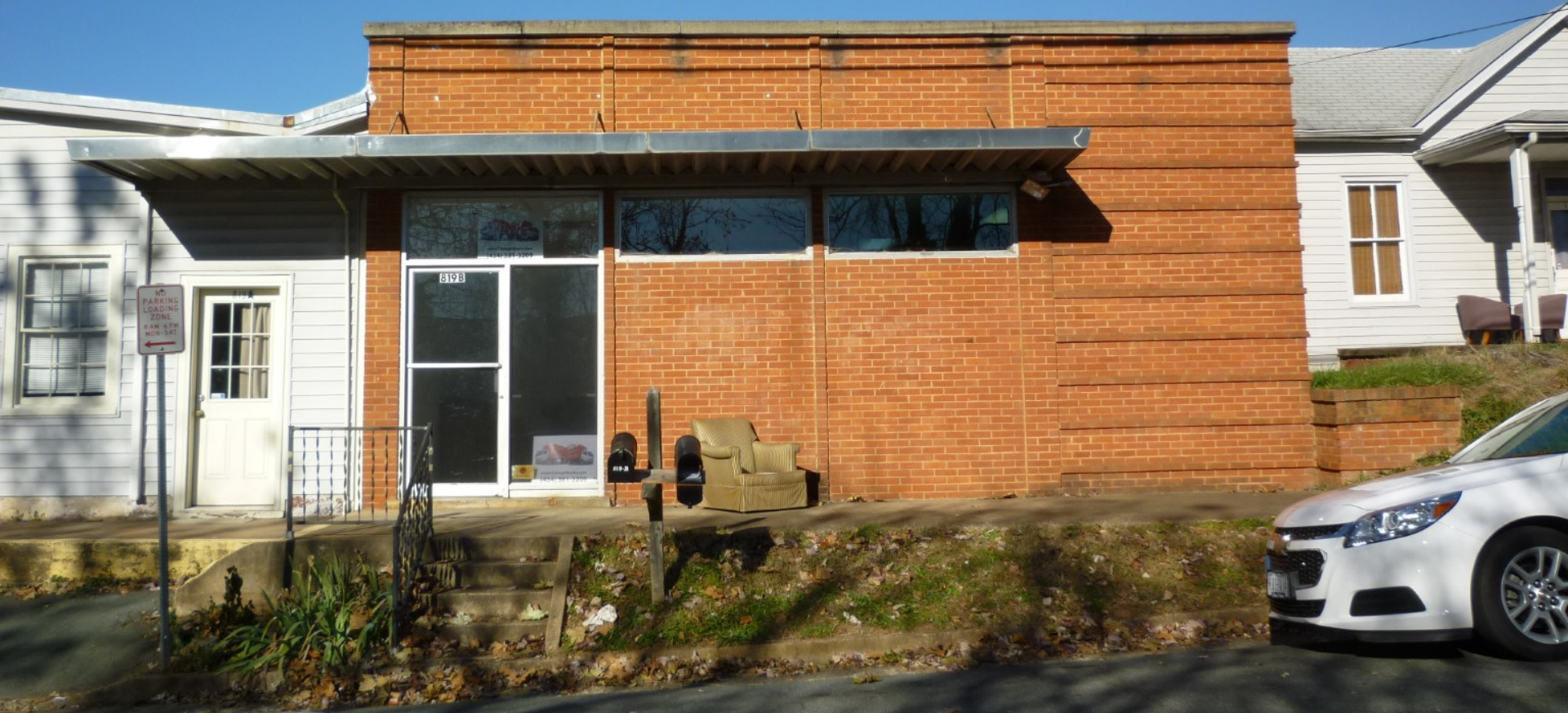
104-5276-0085, Commercial Building, 819 Albemarle Street, east view (Photo taken: 2017)
