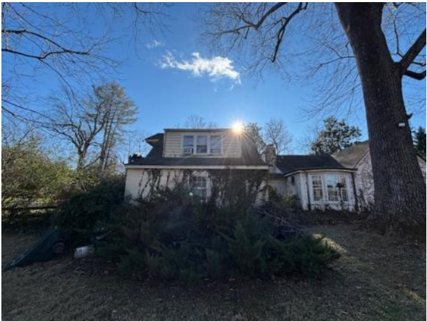
REAR - GARAGE & 1937 PAVILION
