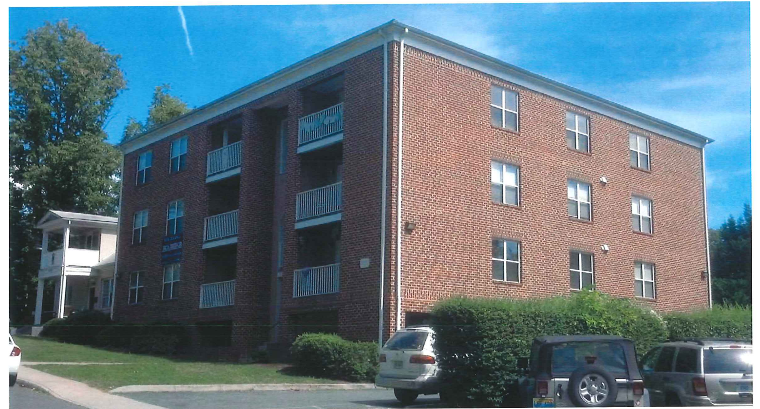
418 17th St. N.W. - 3-story apartment building to remain
