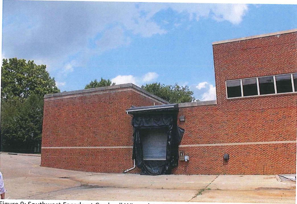
Figure 9: Southwest Façade at Cardwell Wing – late 1990s addition to be removed
