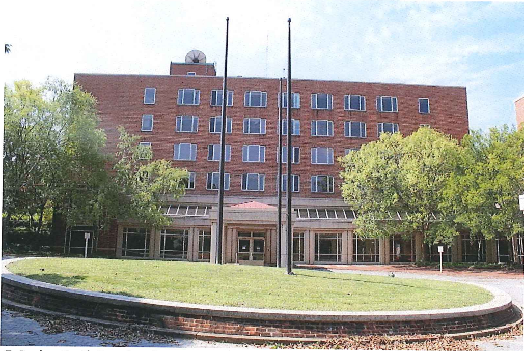
Figure 7: Rucker North Façade – Concourse to be removed
