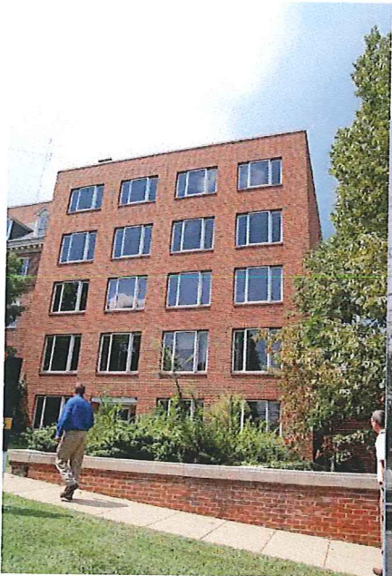
Figure 5: Existing Rucker East Façade
