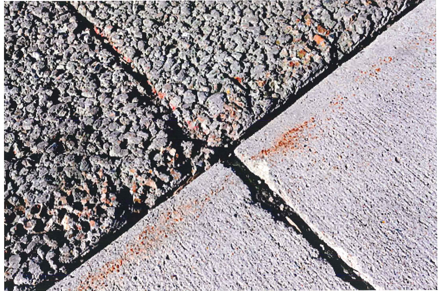
pv-01: porous concrete
