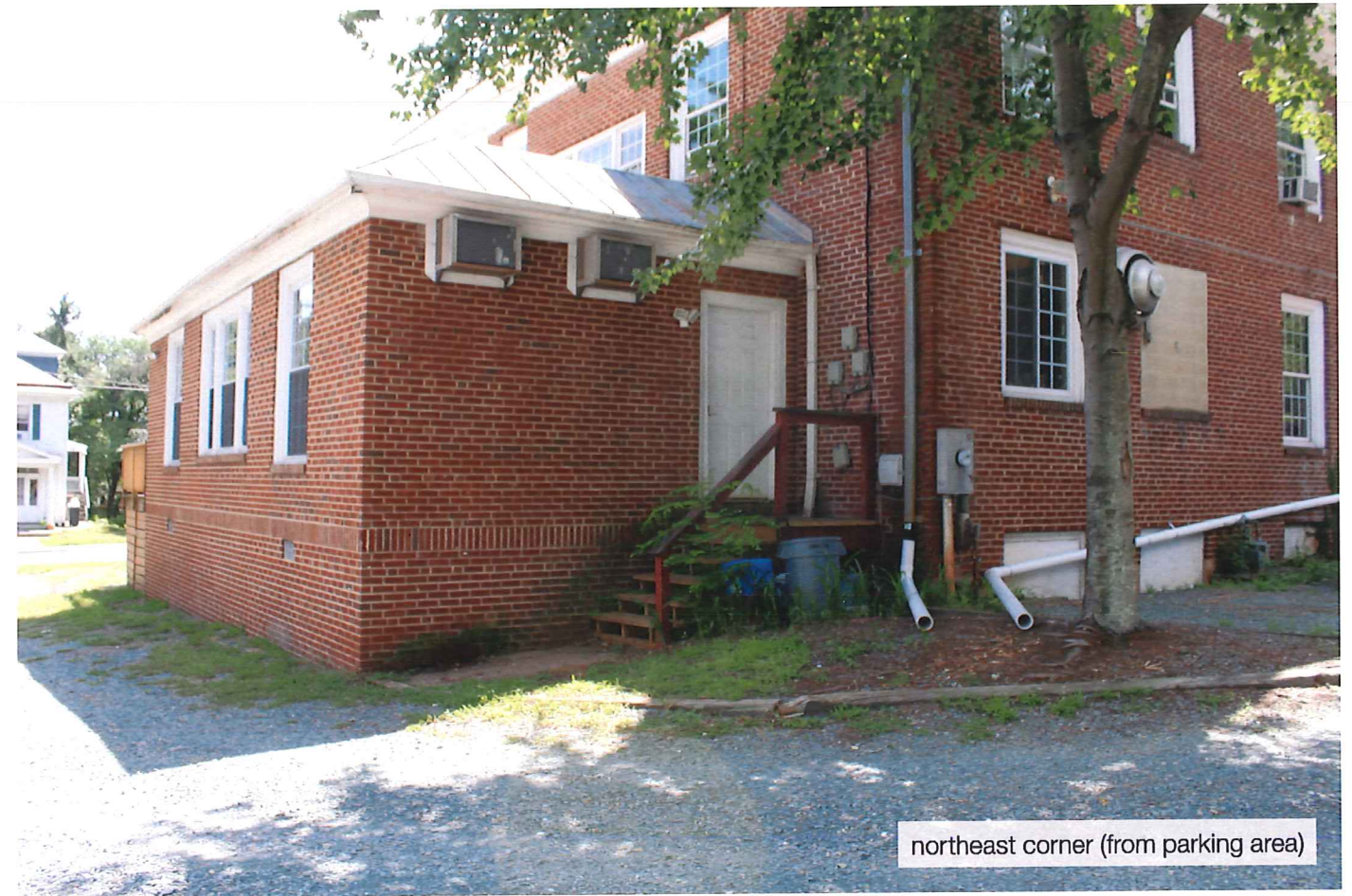
existing retaining wall / deck (from parking area)
