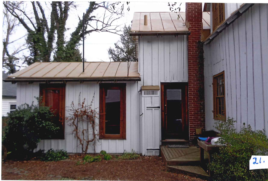
20. 611 Preston Place, Charlottesville, VA Back or NW elevation. Detail of "V" gutter, potential to gush over fence
