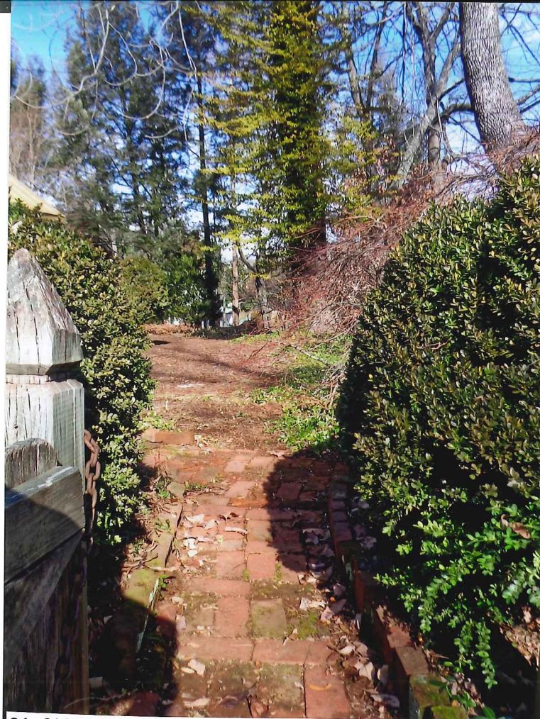
31. 611 Preston Place, Charlottesville, VA Driveway. Detail of gate & walkway leading into front yard. Walk is too narrow for safety, & soldier courses are a trip hazard
