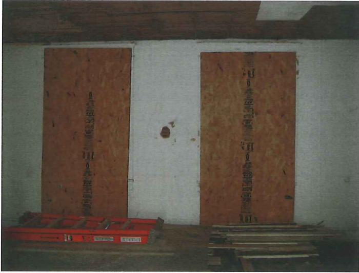
608 Ridge Street Front casement window frames
