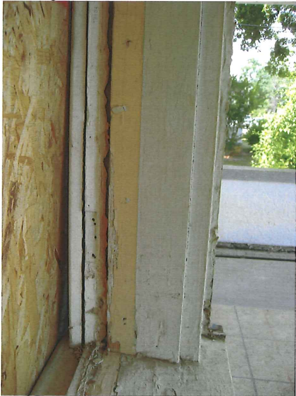
Front casement window frame
