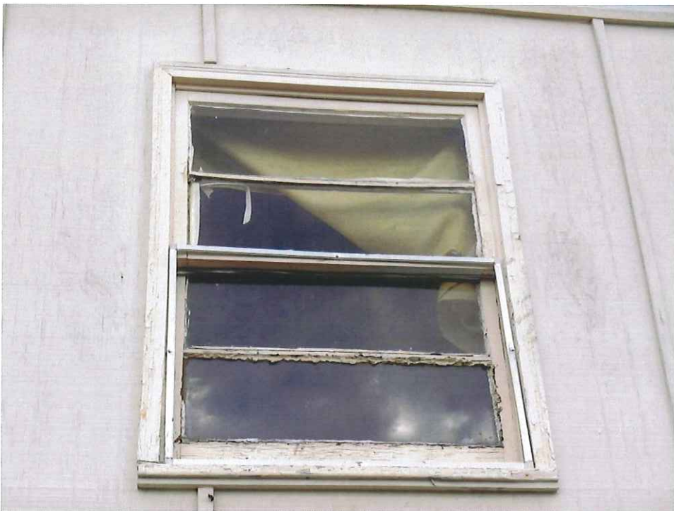
Windows from the 1960's at enclosed back porch to be maintained.
