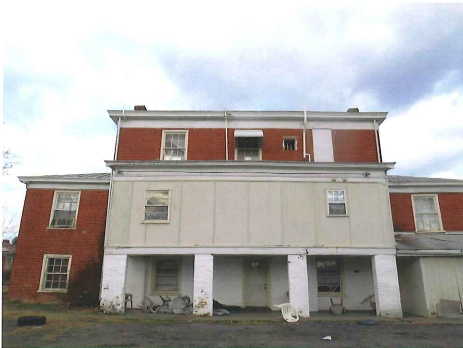
Enclosed back porch to be re-sided.
