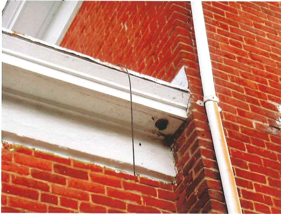
Missing downspouts.
