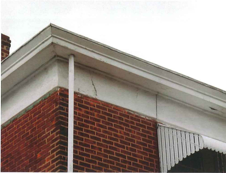
Repair damaged plaster.
