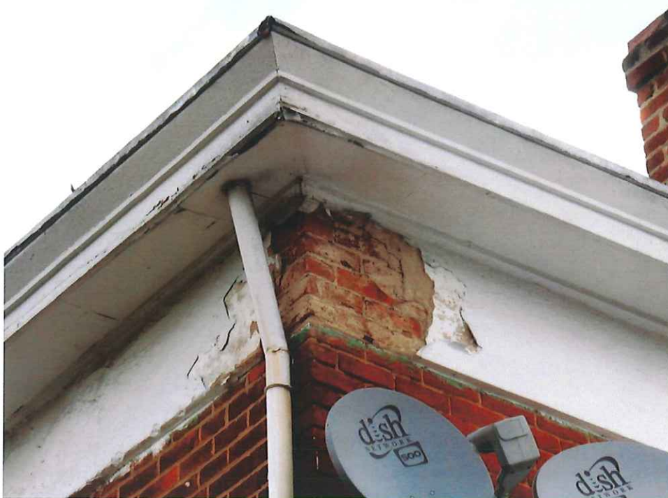
Repair soffit and plaster at 2 nd floor cornice and repaint.
