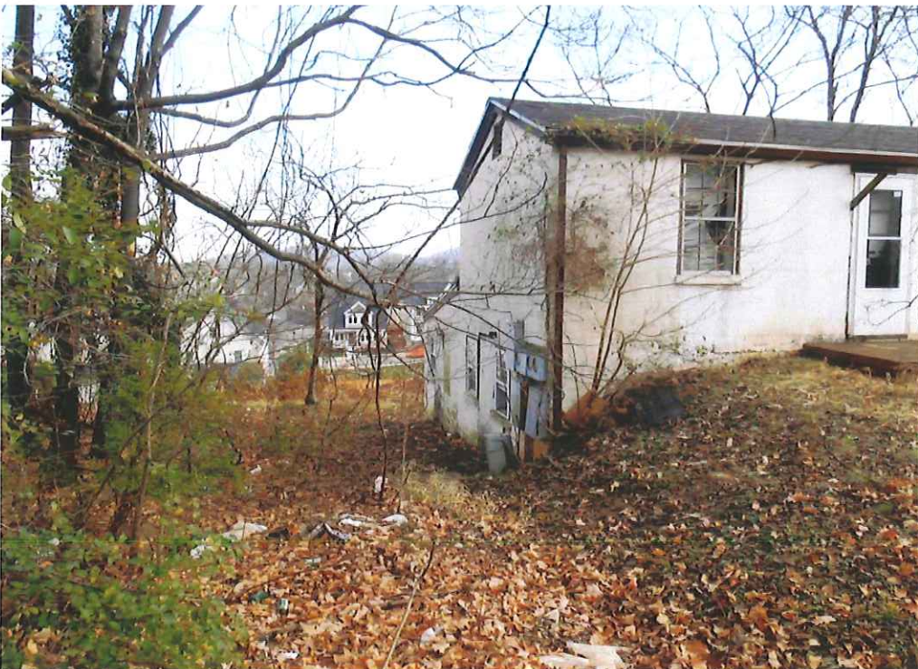
Front NW Corner
