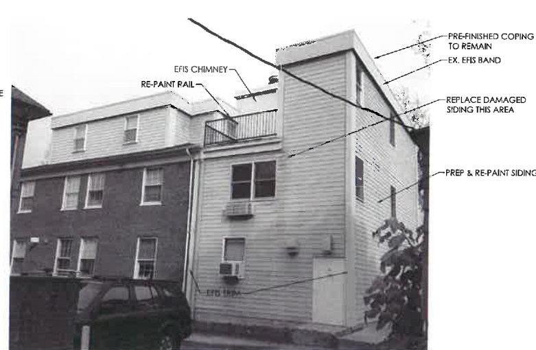
SOUTH ELEVATION - EXISTING SCALE: 1/8" = 1'-0"
