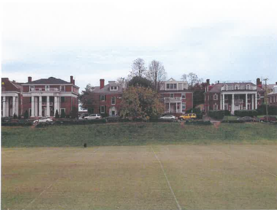
ZTA HOUSE CONTEXT – LOOKING FROM RUGBY ROAD AT ZTA HOUSE
