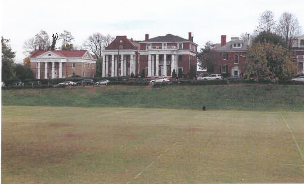
ZTA HOUSE CONTEXT – LOOKING FROM RUGBY ROAD NORTH OF ZTA HOUSE
